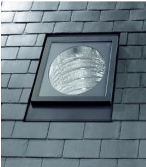
Example of sun tube let into a slate roof
