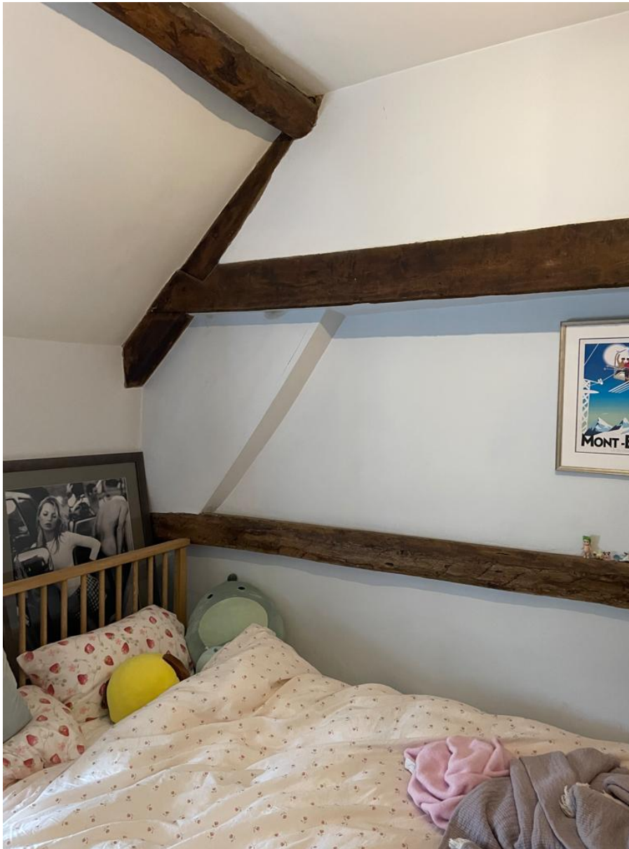
The principal truss within Bedroom 2 with its raised collar is shown above the Mont Blanc picture, the outline of the adjoining lower roof is visible within the plasterwork, and the lower tie is just above the bedhead. Photo from Section AA side of the dividing wall
