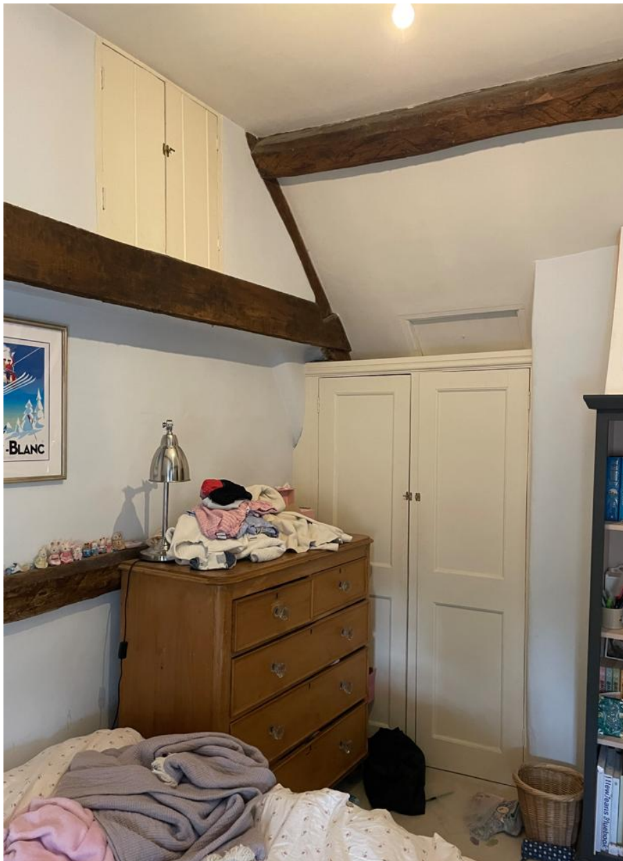
Another photo within Bedroom 2 from Section AA side of the dividing wall, with the lower tie partially concealed by the built in cupboard, the proposed opening is behind the chest-of-drawers. Note this is the cupboard to be copied to form new within Bedroom 1.
