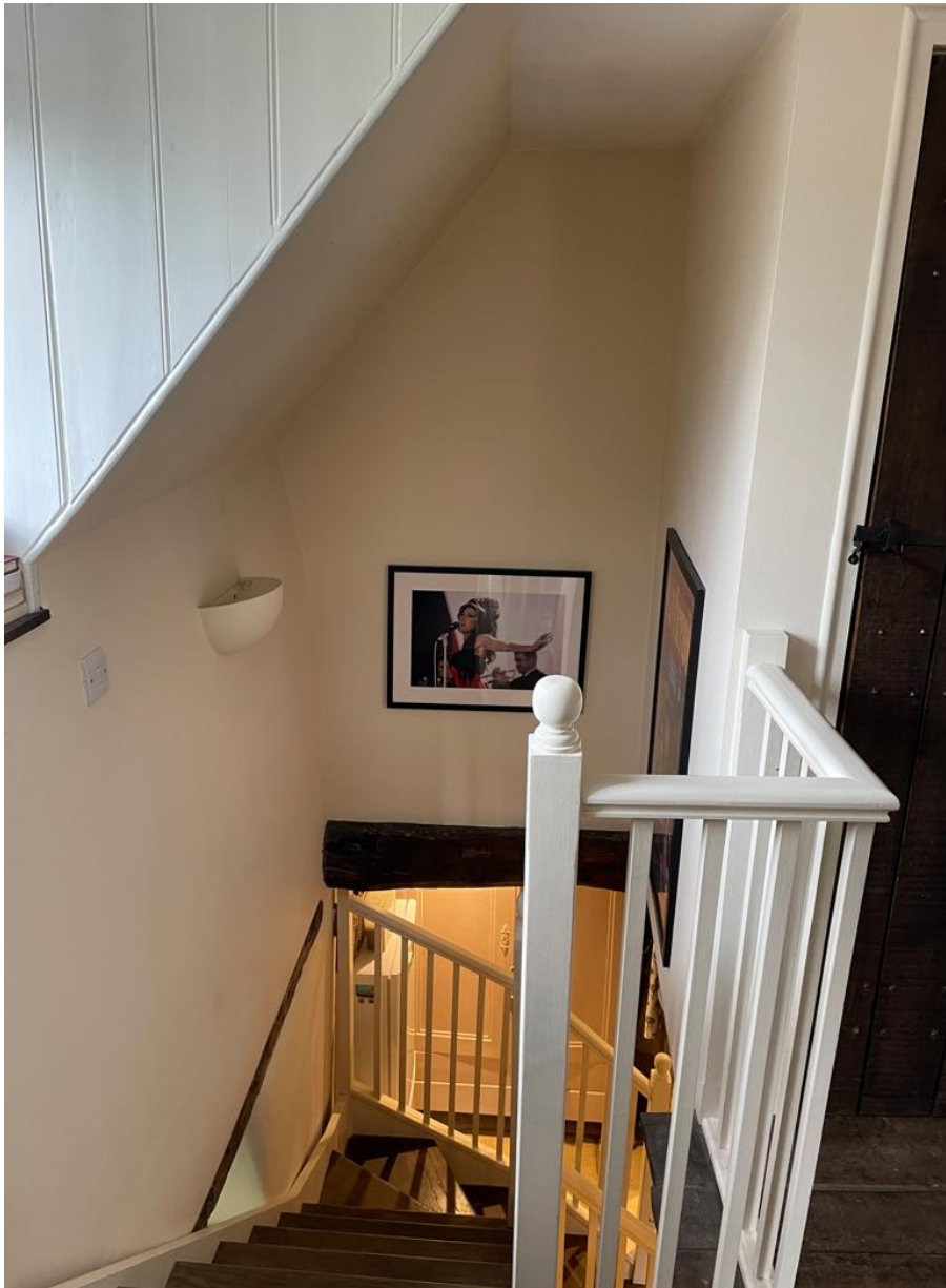
View from Bedroom 1 above kitchen, showing the stairs emerging from the kitchen, and the wall through which the new opening is proposed
