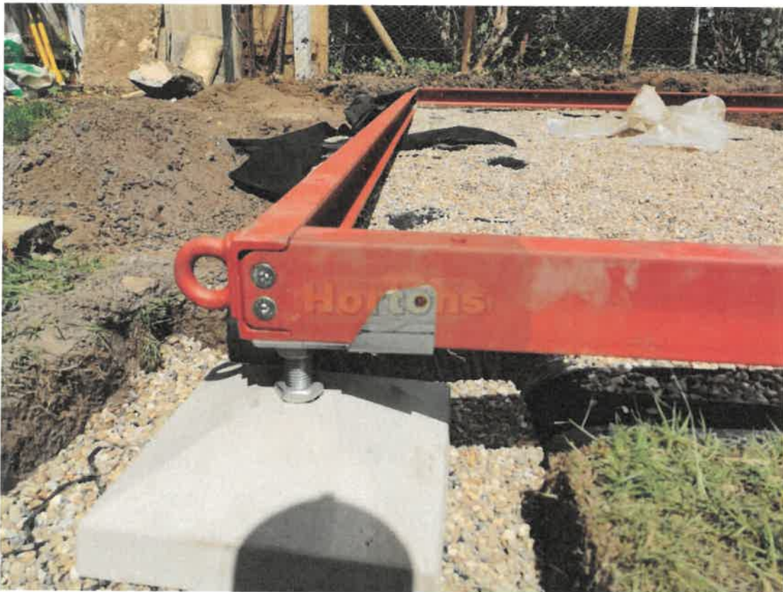
Illustration of proposed structural chassis construction including support pads and lifting eyes.
