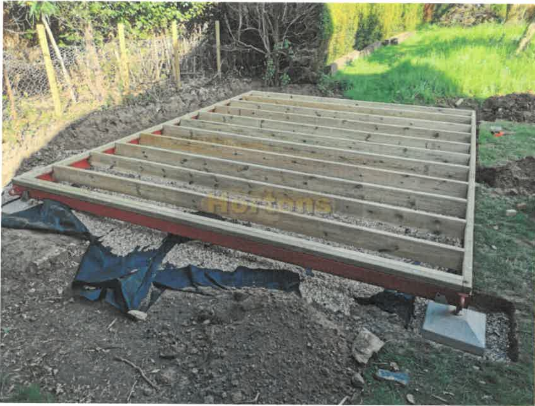
Illustration of proposed structural chassis construction including concrete support pads.
