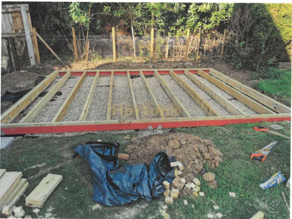
Illustration of proposed structural chassis construction including timber cross members.
