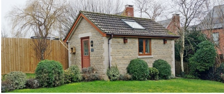
1. General view of existing outbuilding from the rear garden
