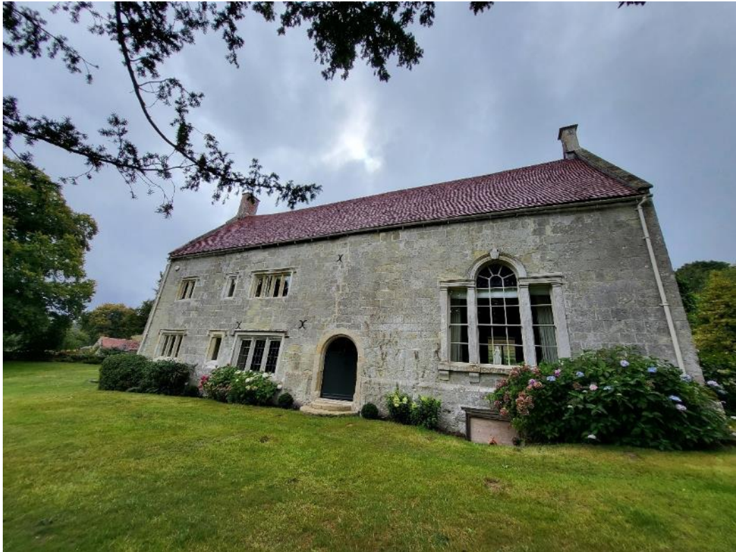
Plate 1: Front (east) elevation of main range
