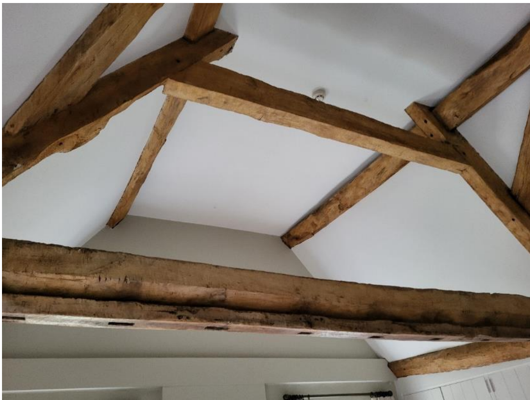
Plate 20: Roof structure in S6, main range
