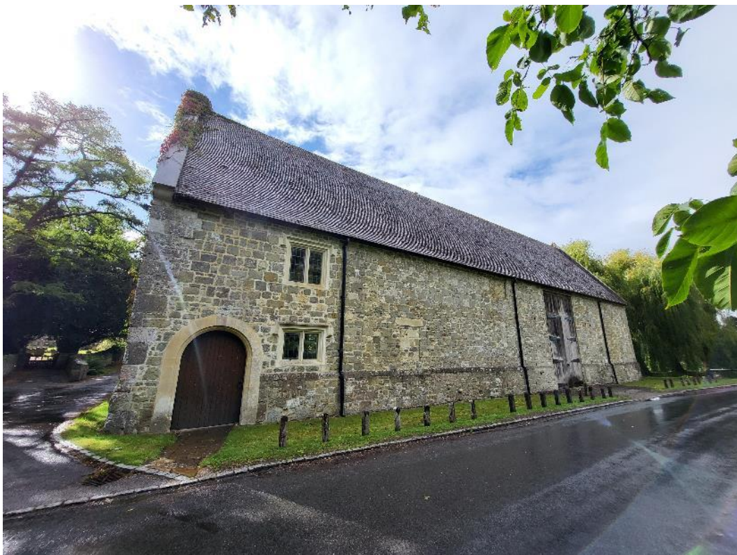
Plate 34: The Grade II* listed Workshop, east elevation onto the road
