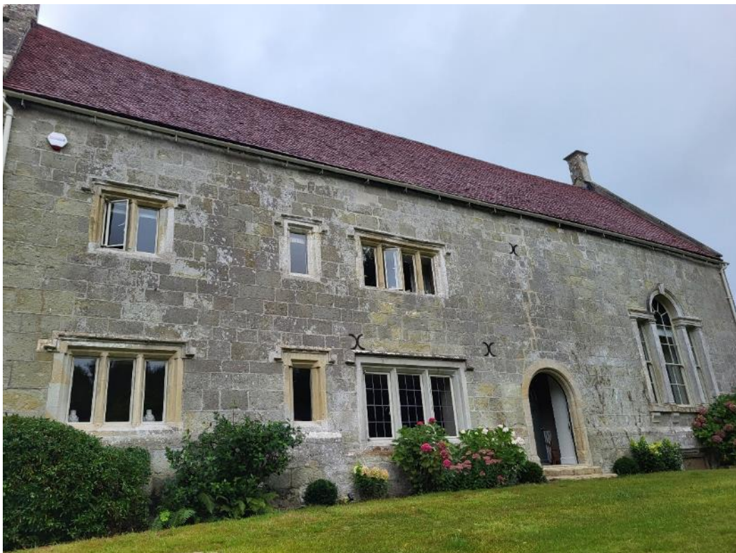
Plate 2: Front (east) elevation of main range
