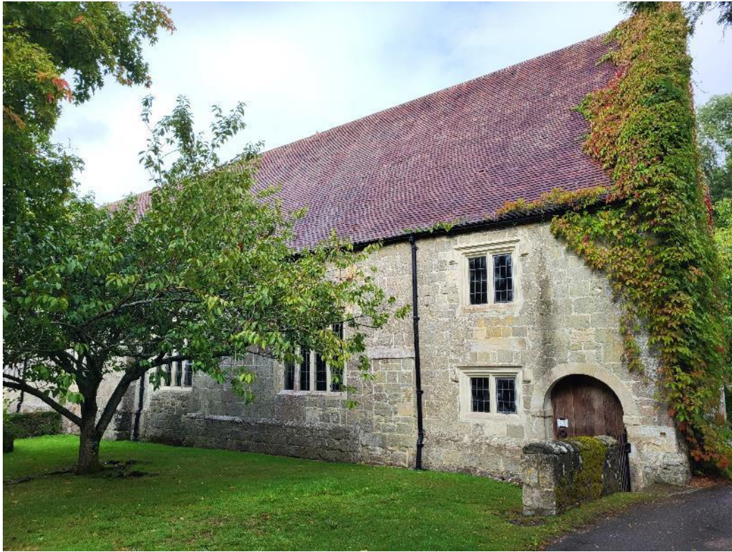
Plate 33: The Grade II* listed Workshop, west elevation facing across Ansty Pond towards the Manor House
