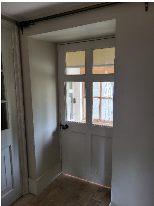
Plate 28: Doorway converted from window opening in north wall of rear wing (G7), opening into link to swimming pool building
