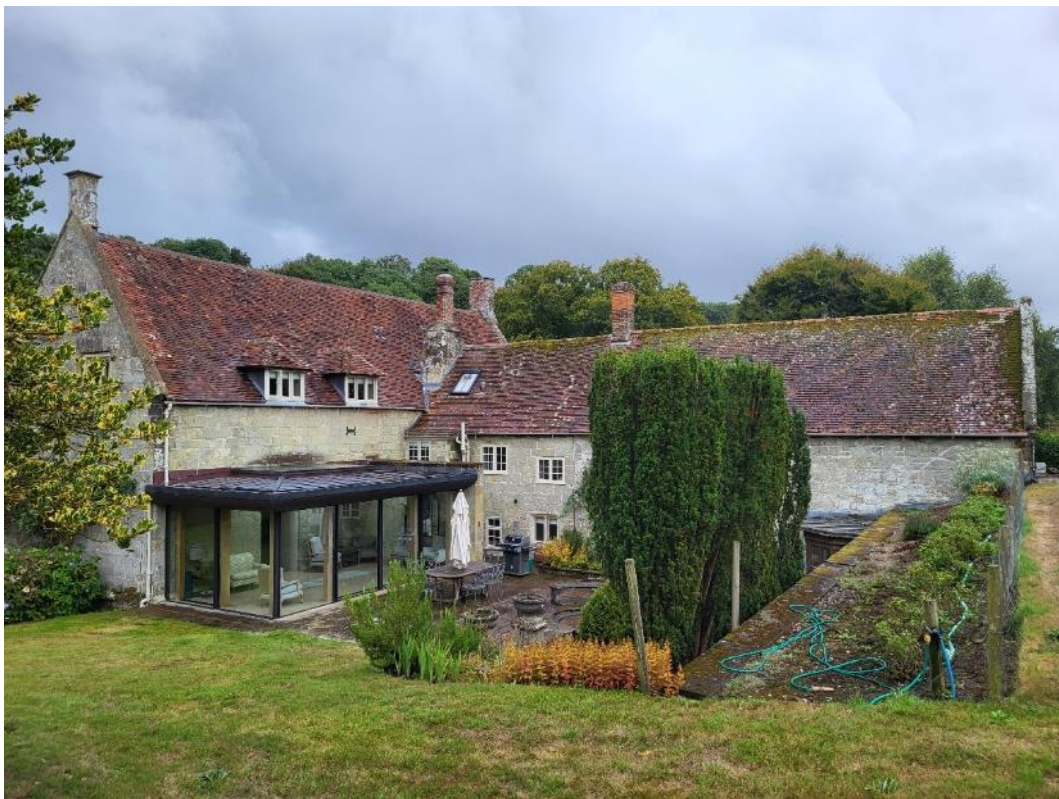
Plate 12: Looking south towards the rear courtyard (roof of swimming pool frontage structure to right)
