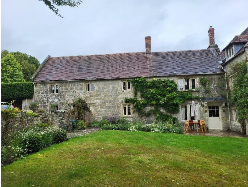
Plate 23: South elevation of rear wing; construction joint between original building (left) and post-1817 infill (right) is aligned with the chimney and change in roof tiles
