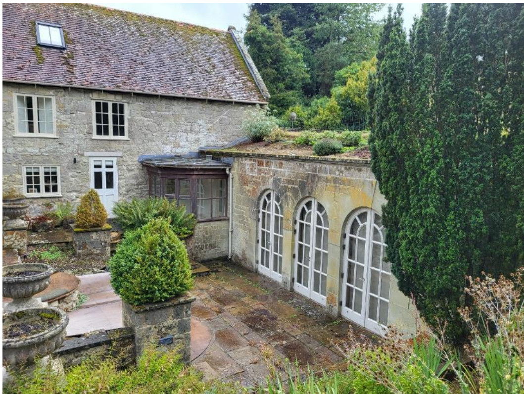
Plate 30: Looking towards linking structure between rear wing and swimming pool
