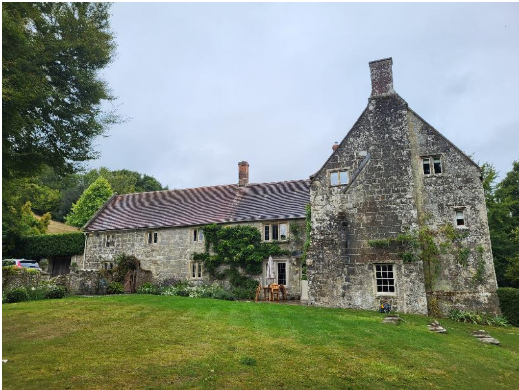
Plate 22: South elevation of rear wing and gable end of main range
