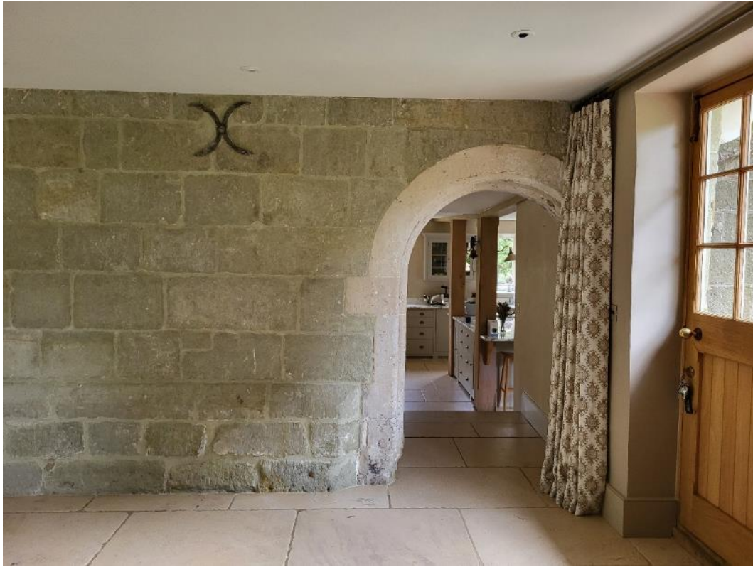
Plate 3: Rear wall of front range, now internalised within post-1817 extension connecting main range and rear wing, with formerly external round-arched opening
