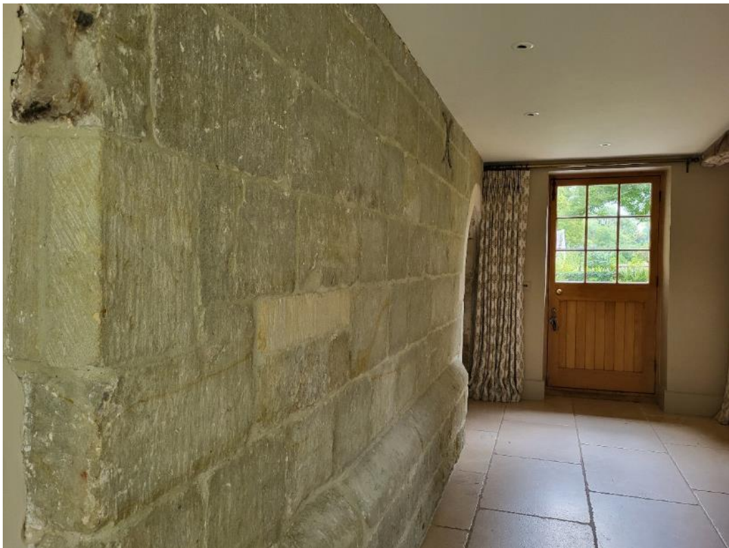
Plate 4: Rear wall of front range; note plinth/base moulding
