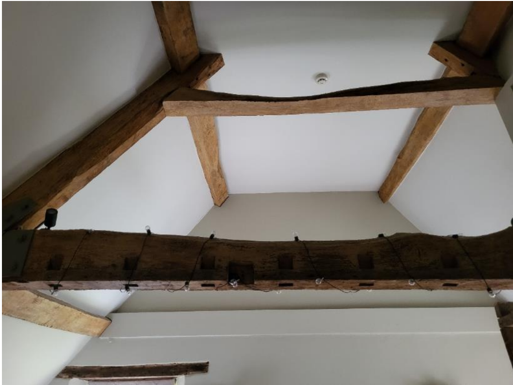
Plate 19: Roof structure in S2, main range
