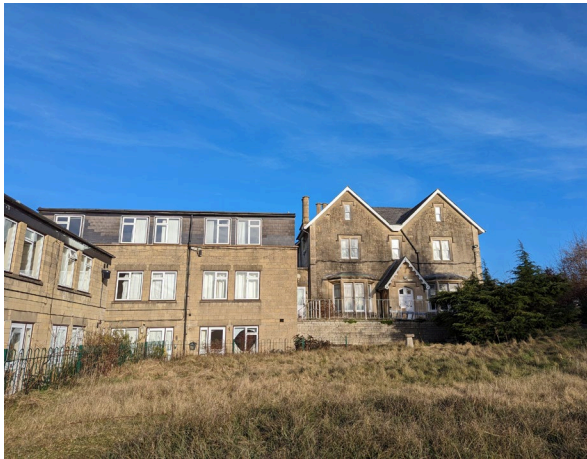
Plate 1: Lenora House, southern elevation with the original house to the east and flat roof extension to the west
