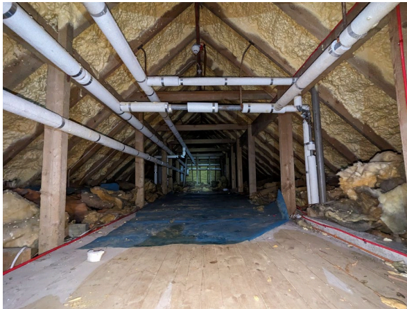
Plate 5: northern roof void, where a dead common pipistrelle bat was found
