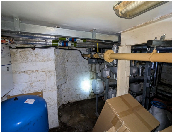
Plate 7: Basement of Lenora House
