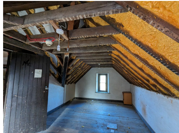
Plate 6: southern roof void of Lenora House
