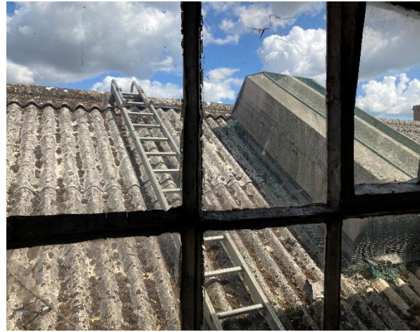
Figure 11 - The roof of the building
