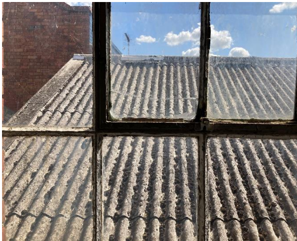
Figure 11 - Roof of the main building.
