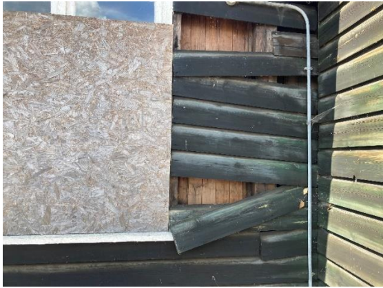
Figure 15 – Scott's Gym, cavity wall.
