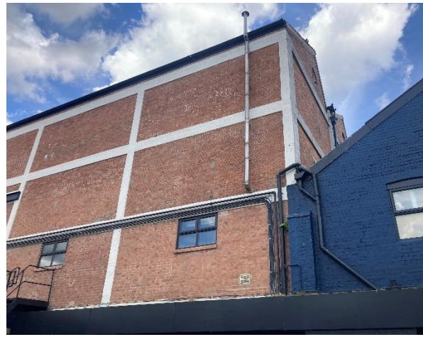
Figure 12 - Condition of the external brickwork of the main building.
