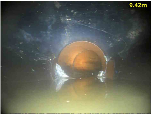
4, 00:01:26, 9.42 m Finish node, manhole, reference: MH6
