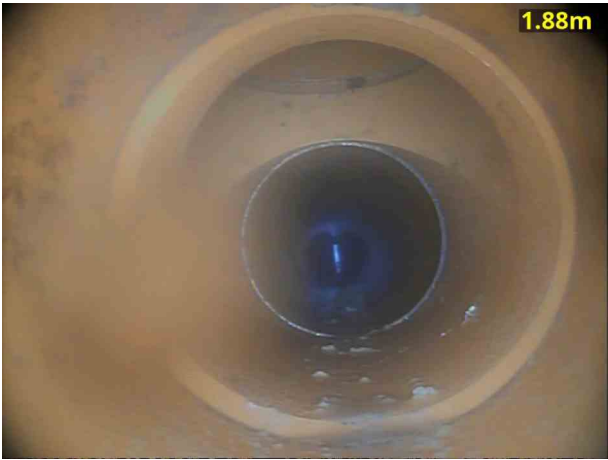
2, 00:00:22, 1.88 m Junction at 12 o'clock, 100mm dia
