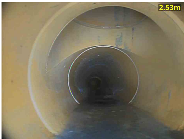
3, 00:00:52, 2.53 m Junction at 12 o'clock, 100mm dia
