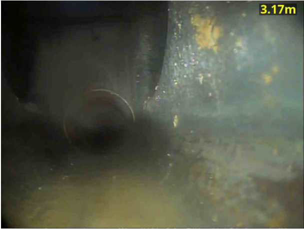
4, 00:00:38, 3.17 m Finish node, manhole, reference: MH16
