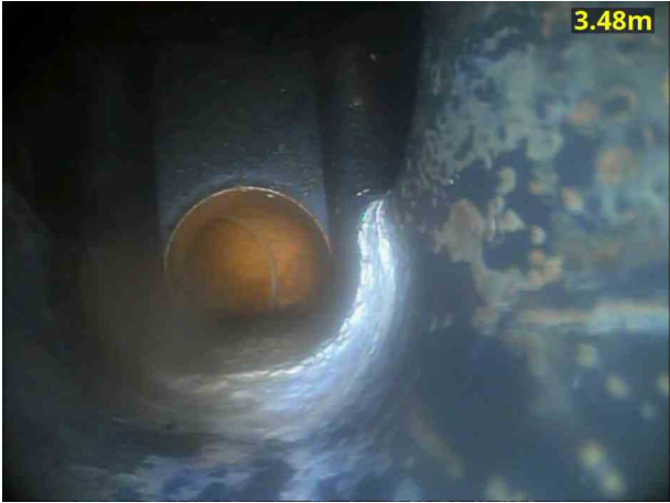
4, 00:00:40, 3.48 m Finish node, manhole, reference: MH17
