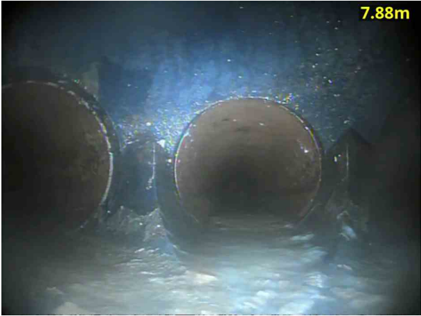
4, 00:01:09, 7.88 m Finish node, manhole, reference: MH11
