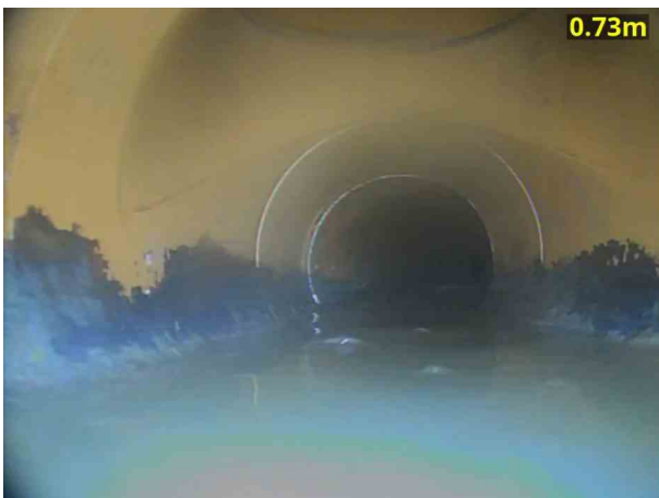
3, 00:00:30, 0.73 m Junction at 12 o'clock, 100mm dia
