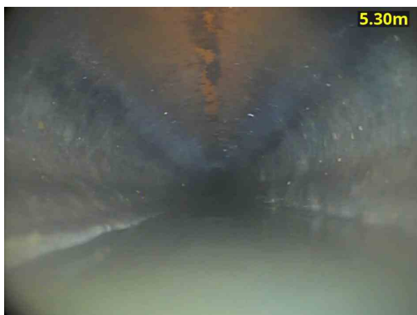
5, 00:00:53, 5.30 m Water level, 10% of the vertical dimension
