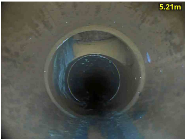
3, 00:00:48, 5.21 m Junction at 12 o'clock, 100mm dia
