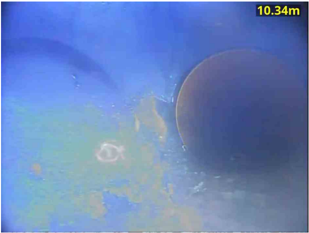
7, 00:01:39, 10.34 m Finish node, manhole, reference: MH10
