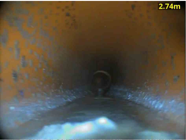
3, 00:00:31, 2.74 m Water level, 10% of the vertical dimension
