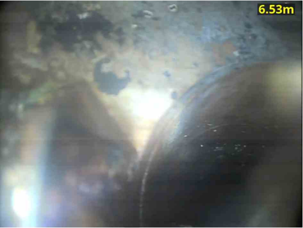
3, 00:01:08, 6.53 m Finish node, manhole, reference: MH7
