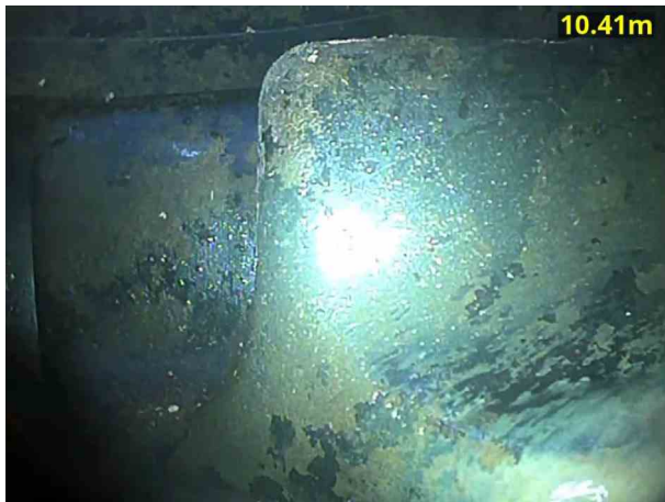
5, 00:01:28, 10.41 m Finish node, manhole, reference: MH3
