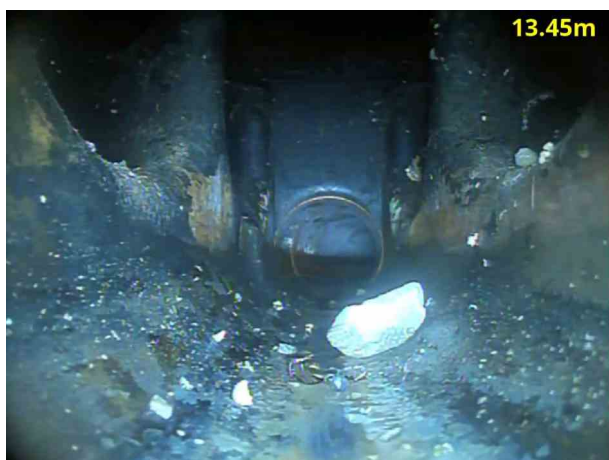
5, 00:01:46, 13.45 m Finish node, manhole, reference: MH14
