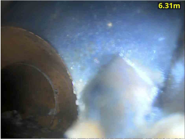
4, 00:00:45, 6.31 m Finish node, manhole, reference: MH18
