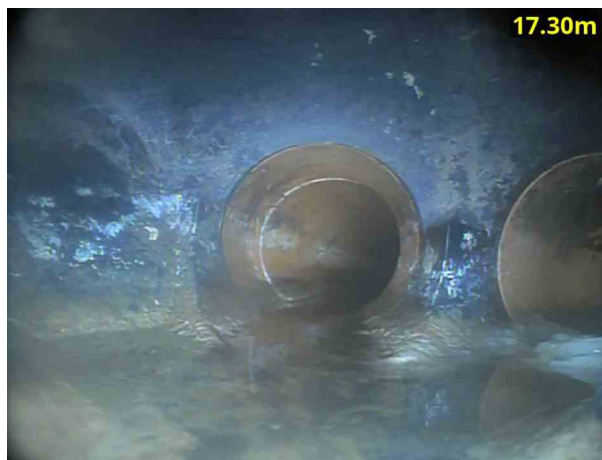
6, 00:02:20, 17.30 m Finish node, manhole, reference: MH8
