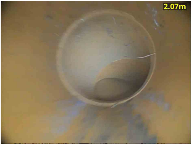
2, 00:00:22, 2.07 m Roots, fine at joint
