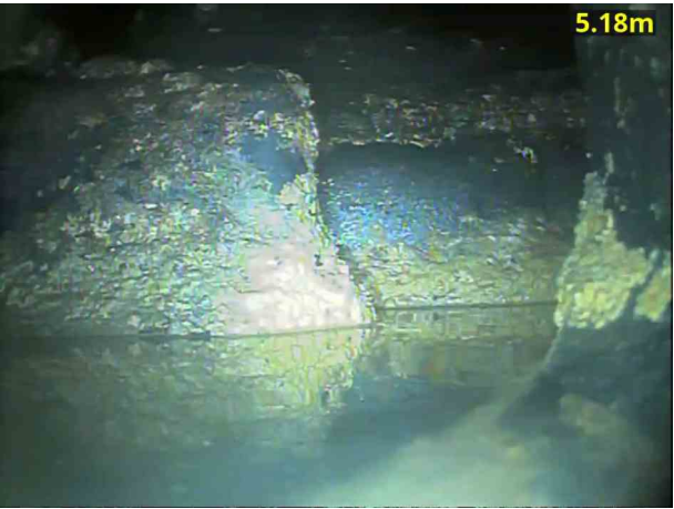
3, 00:00:43, 5.18 m Finish node, manhole, reference: MH12
