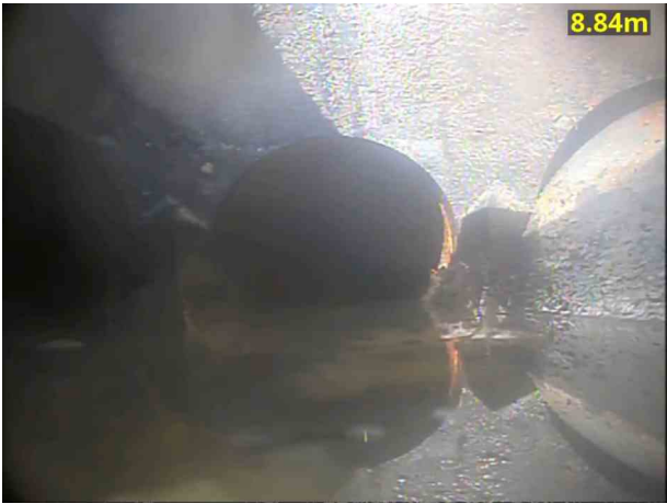
8, 00:01:37, 8.84 m Finish node, manhole, reference: MH5
