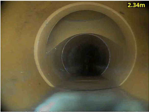
2, 00:00:27, 2.34 m Junction at 12 o'clock, 100mm dia
