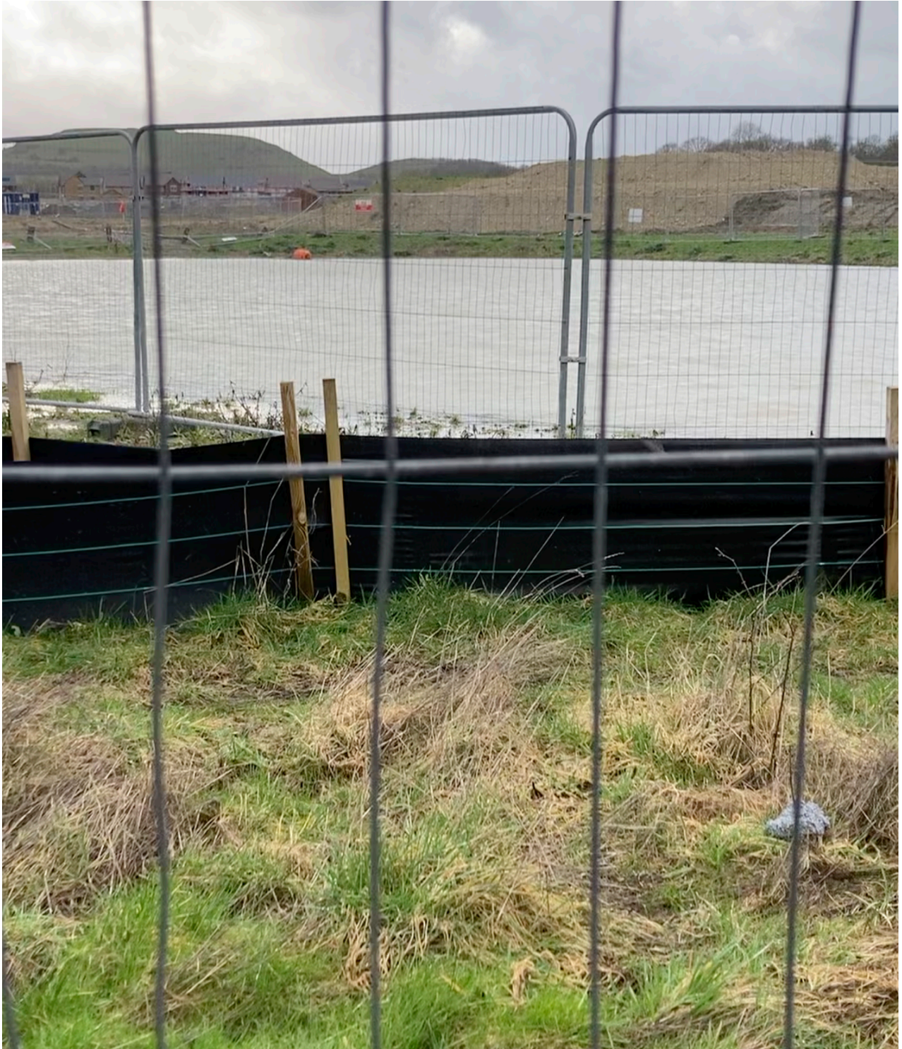
Above: Water in the attenuation pond is flooding, requiring extra barricading.
