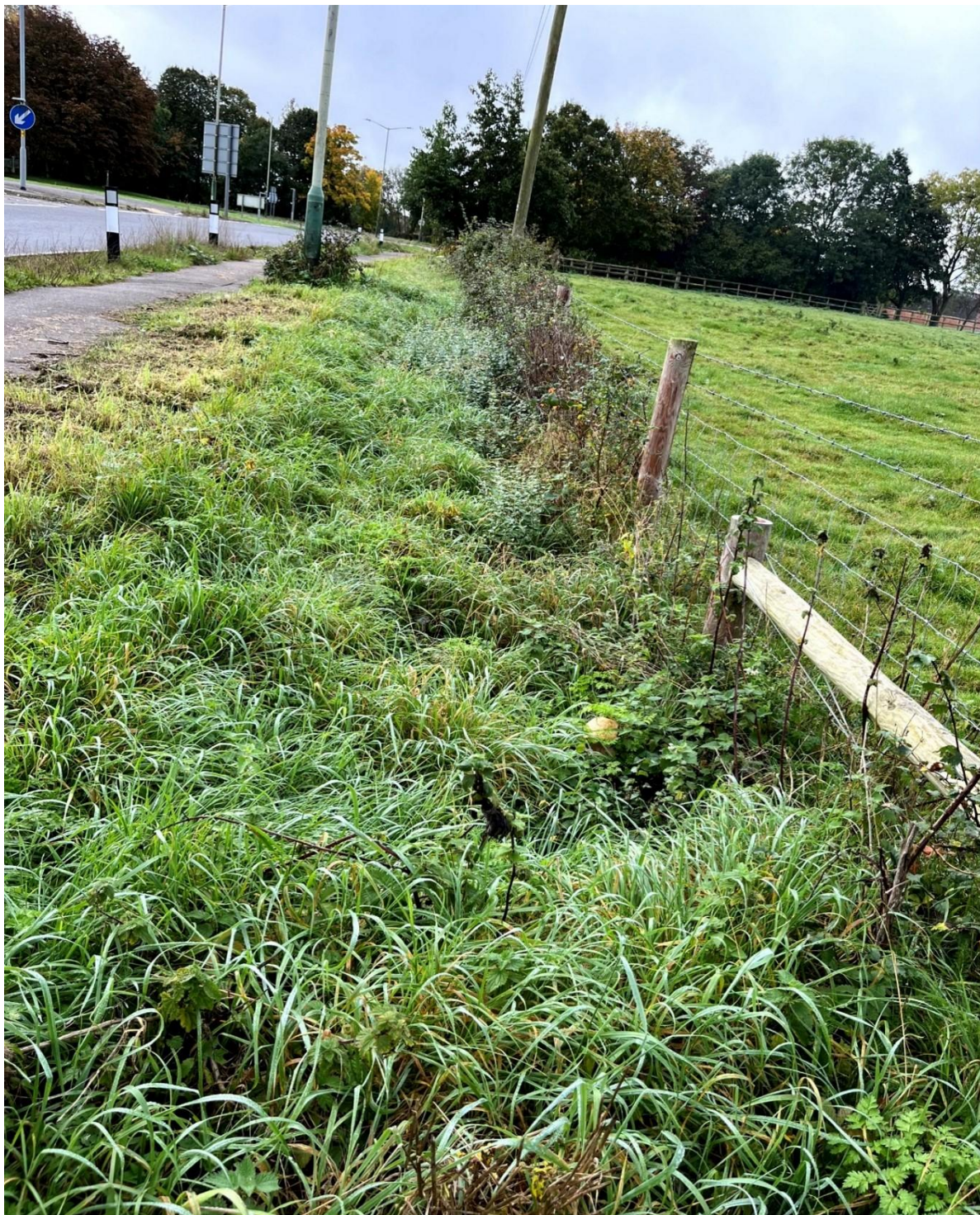
Figure 3.5: Photograph of the Eastern Highway Ditch
