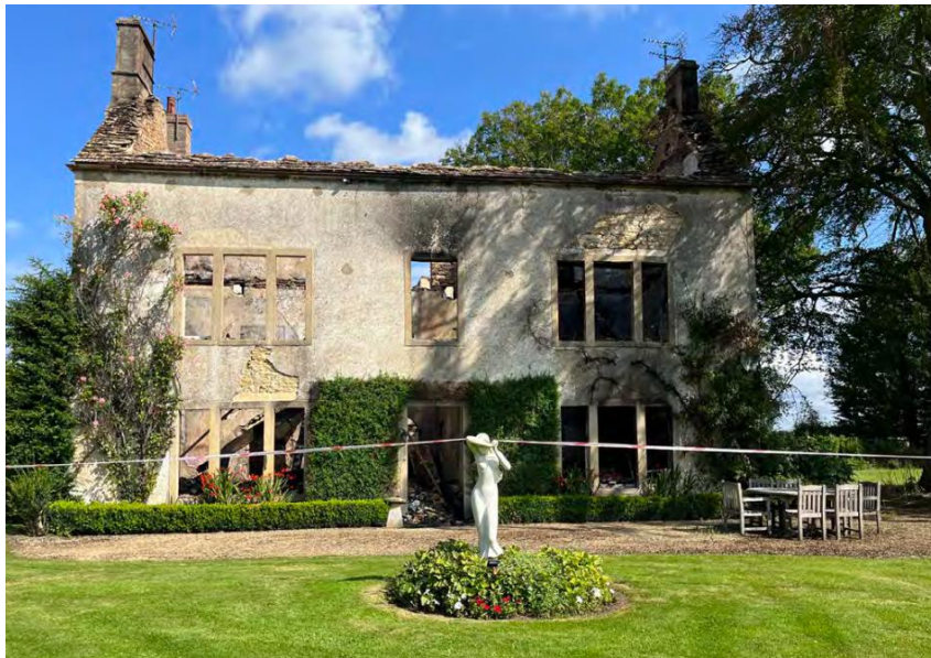
Front Elevation Photo – taken from the Heritage Statement
