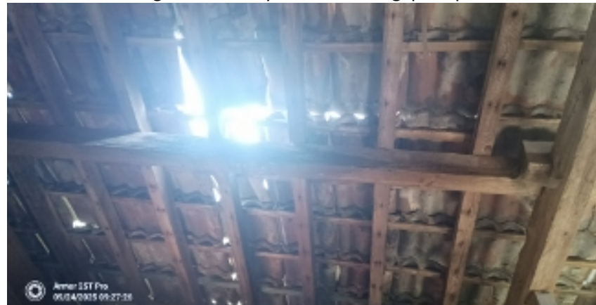
Photo 10. Showing un-lined clay tile roof with gaps in places
