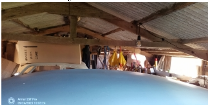
Photo13. Interior of large timber shed
