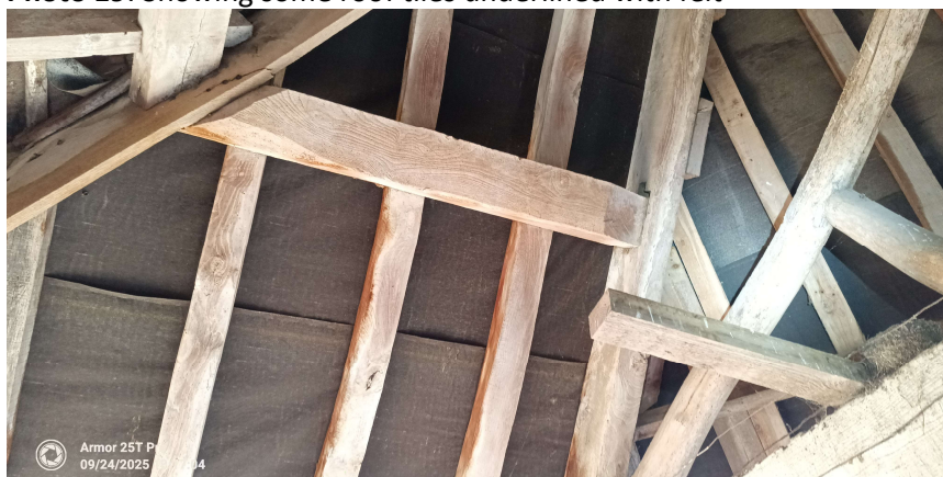
Photo 19. Showing some roof tiles underlined with felt
