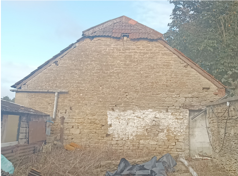
Photo 12. East gable end of Cart Shed with some holes in the laid stone
