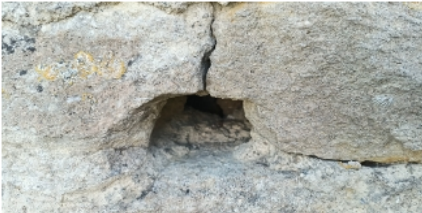
Photo 12. East gable end of Cart Shed with some holes in the laid stone
