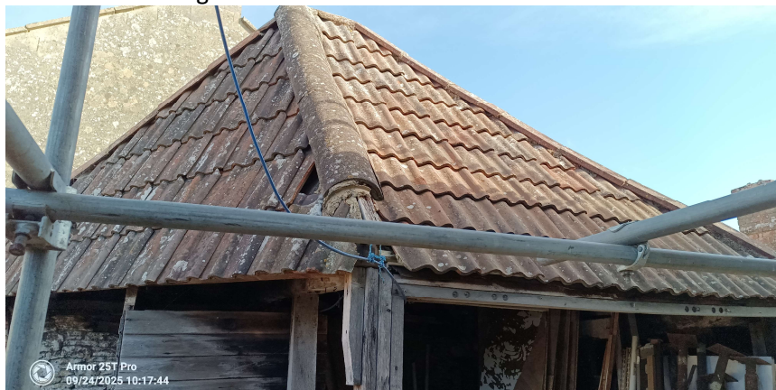
Photo 19. Showing some roof tiles underlined with felt
