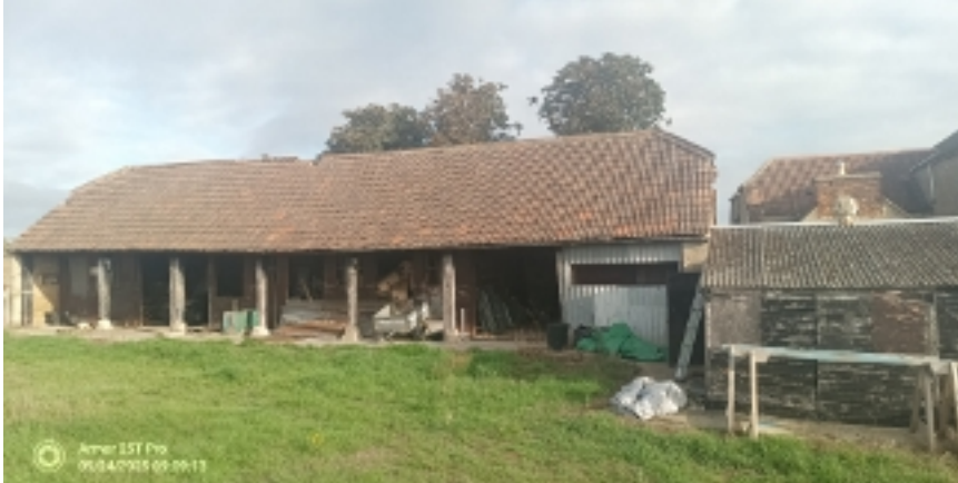
Photo 9. Showing inside of part of the cart shed
