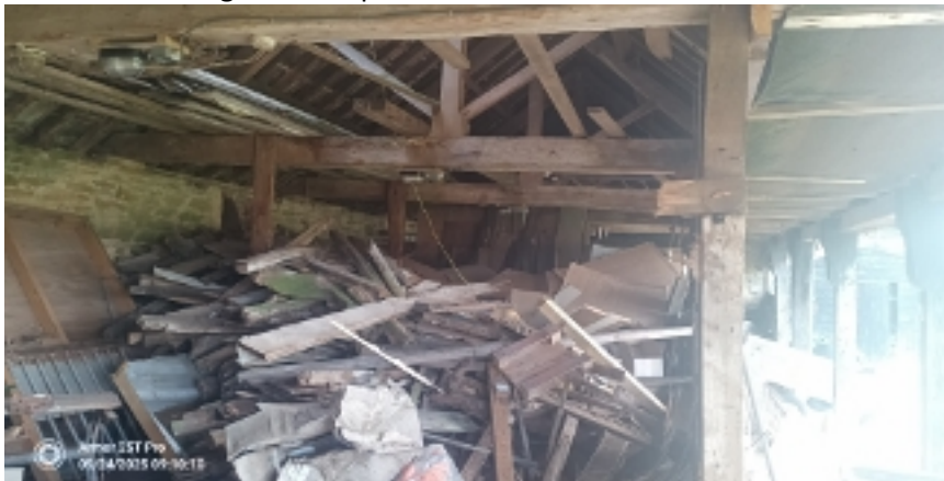
Photo 10. Showing un-lined clay tile roof with gaps in places
