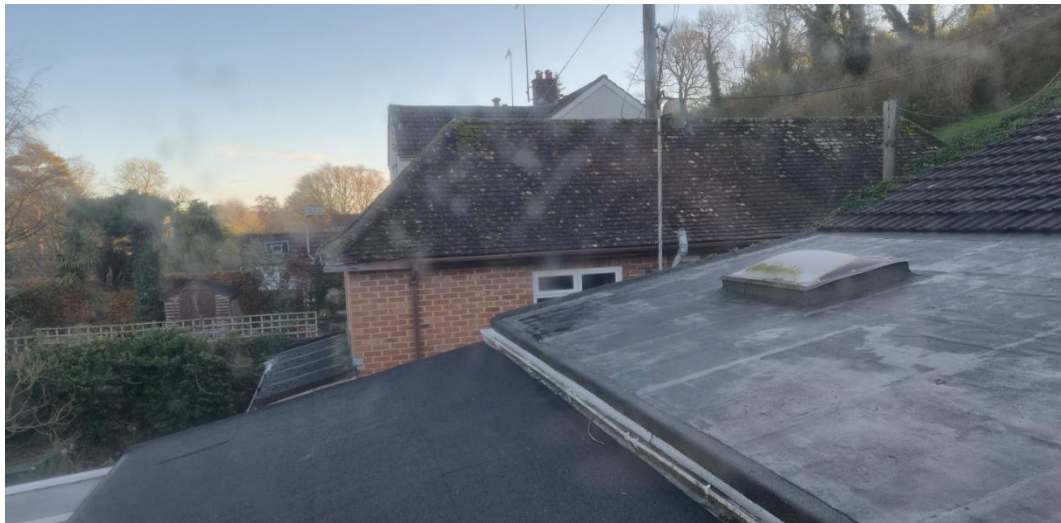
Existing neighbouring windows are blocked by the current dwelling at Cherry Bank
