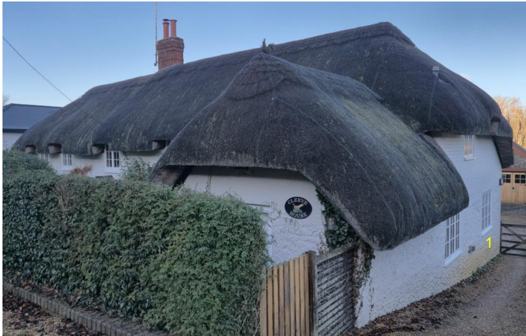
Windows on the side of Cleeves House
