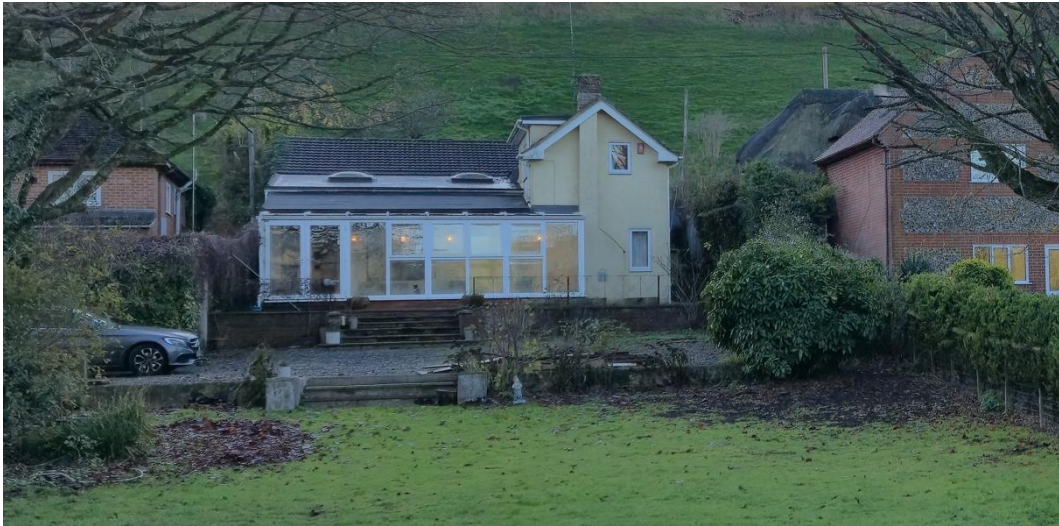
Existing rear elevation of the current dwelling to be demolished
