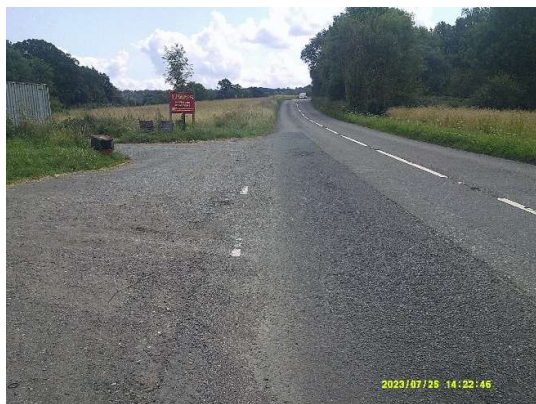
Photo 3: Site access looking southwards
