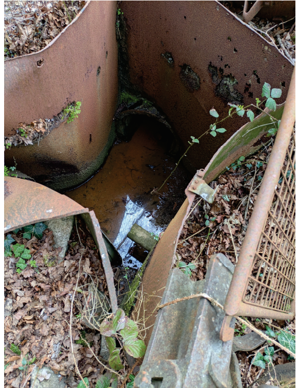
Existing chamber on piped ditch (S12)
