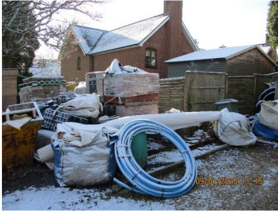
Photo 7: Area of site where new driveway and garage/office building will be constructed.
