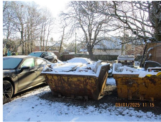
Photo 8: Area of site where new driveway and garage/office building will be constructed.
