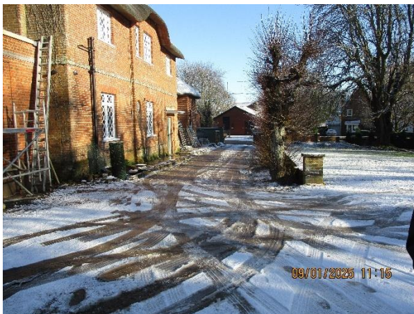
Photo 4: Main house and driveway.
