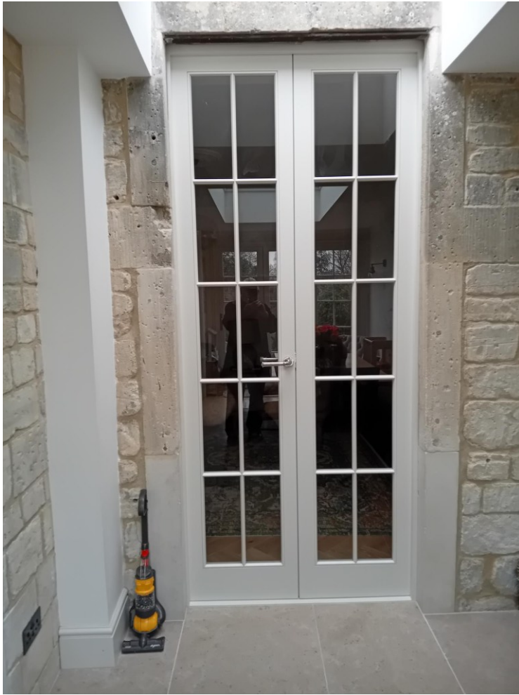
THE DOORS REPLACING WINDOW
