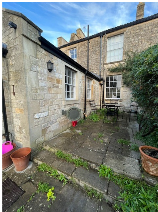
WINDOW PRIOR TO EXTENSION BEING BUILT
