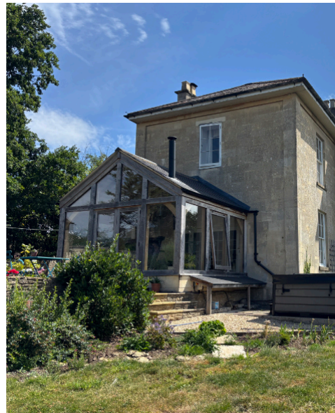
Modern timber conservatory (west elevation).
