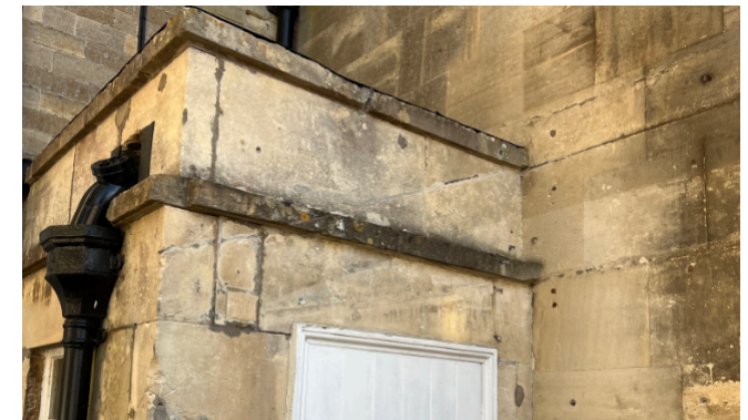
Fig 2. Single storey rear addition with historic evidence of lean-to structure.
