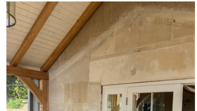
Fig 3. Existing conservatory with historic evidence of pitched roof structure.
