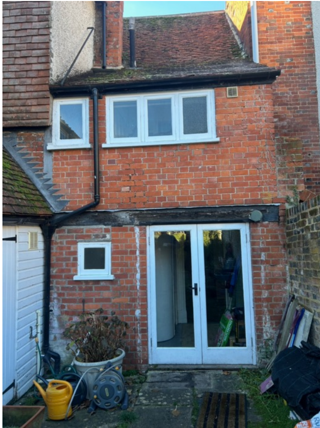
Photo 3 View of existing more modern brickwork to the rear
