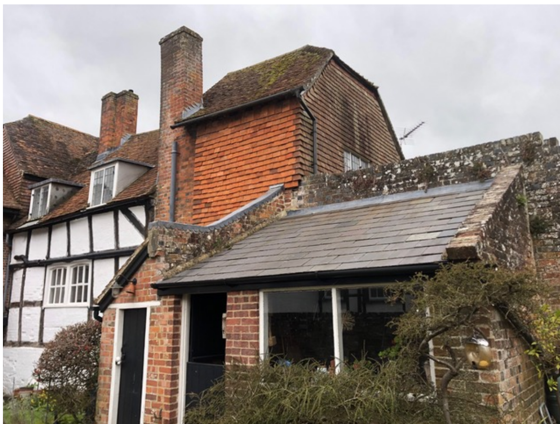
Photo 5 - View of the side elevation chimneys
