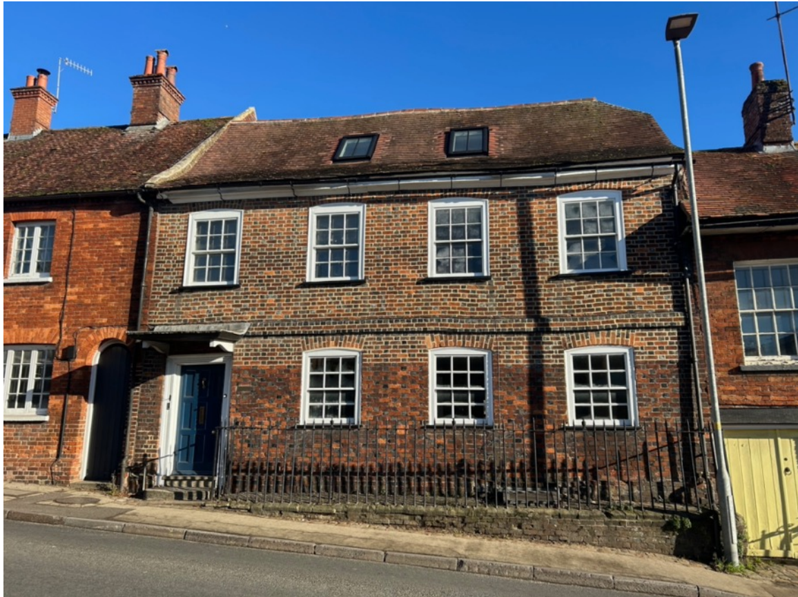
Photo 1 - View of the front elevation from Barn Street
