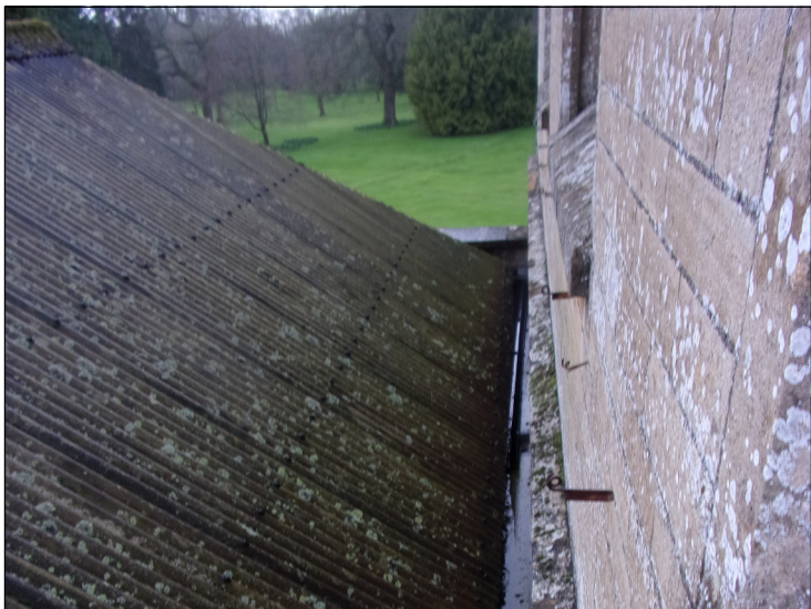
VIEW OF ROOF VALLEY WALL ABUTMENT
