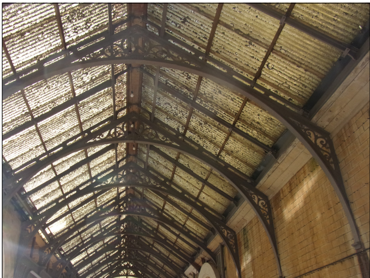
INTERNAL WESTERN VIEW OF ROOF
