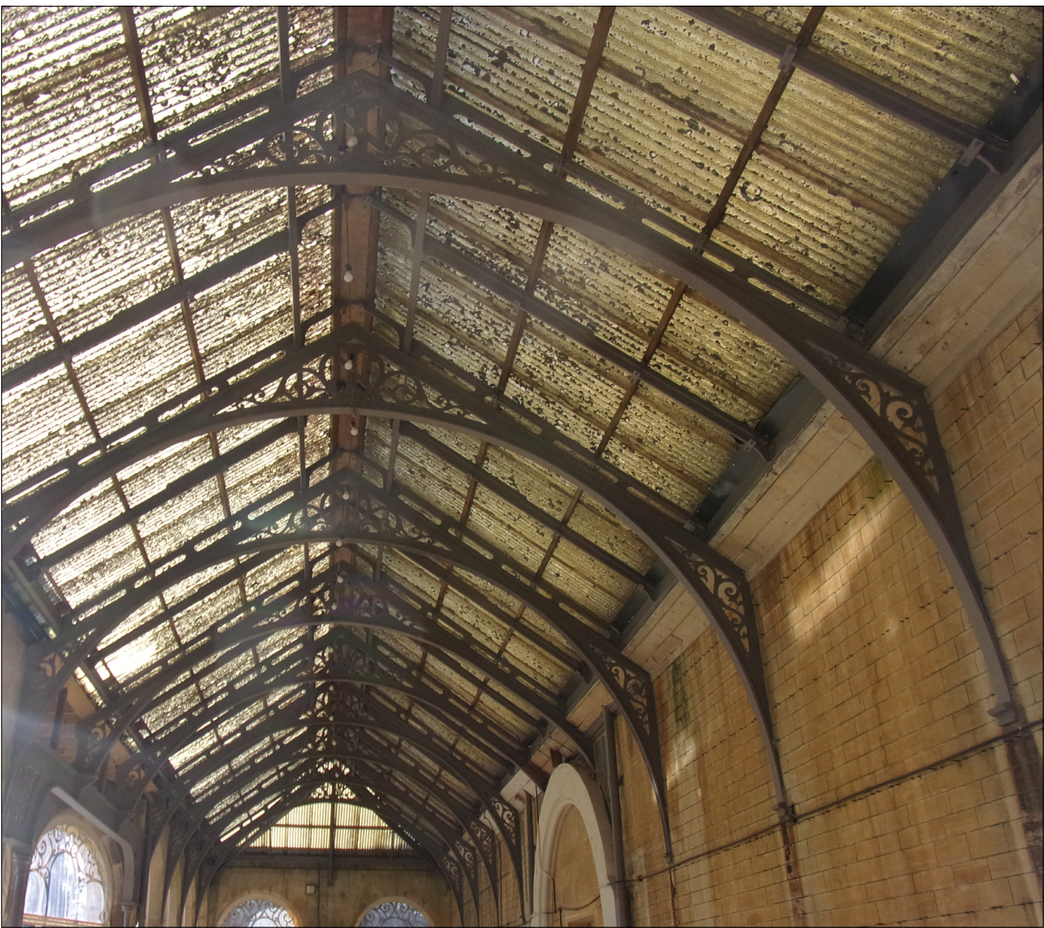
PHOTO INDICATING CORRUGATED FIBREGLASS ROOF SHEETING
