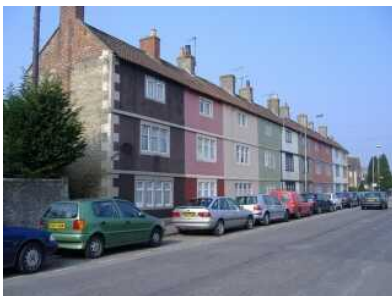
No. 87-105 - 3 storey terrace
