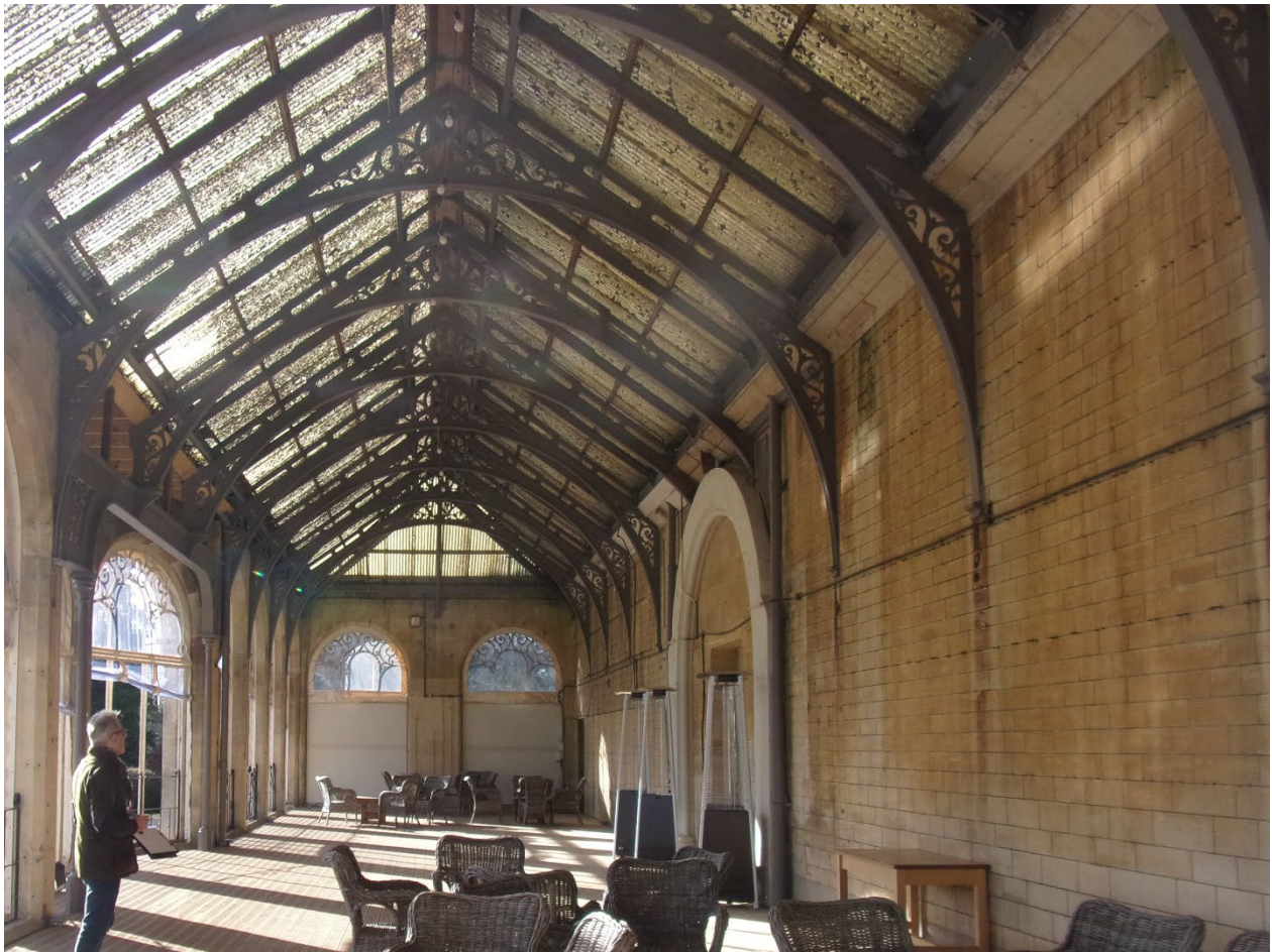
Internal view of The Orangery indicating the roof structure and corrugated roof covering
