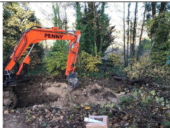
Plate 11 – View SE of lower terrace
