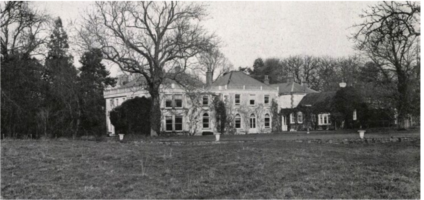
Image from the south of Great Somerford Manor House from Country Life 5 July 1919
