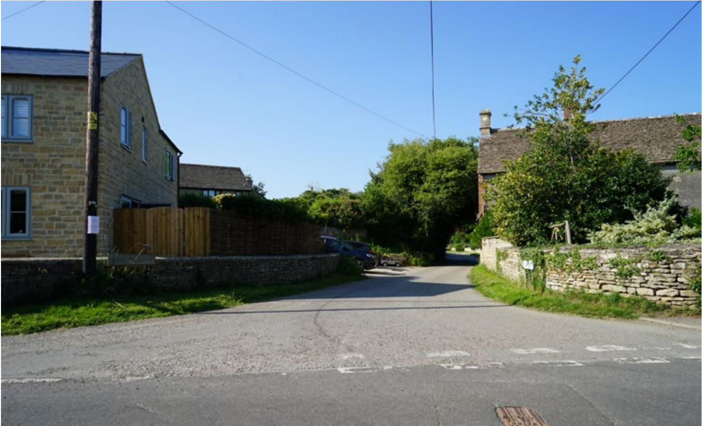
7. One of the series of secondary lanes that help to establish the sense of a highway hierarchy – principal lane, secondary lane and then tertiary 'spurs'.
