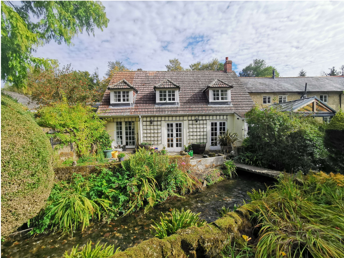
Photograph 02, Rear elevation as existing.
