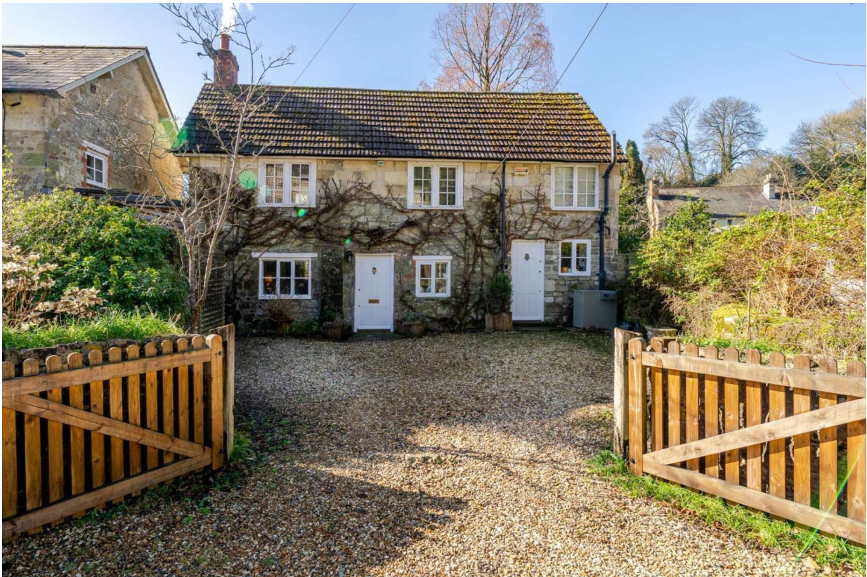
Photograph 01, Front elevation as existing.
