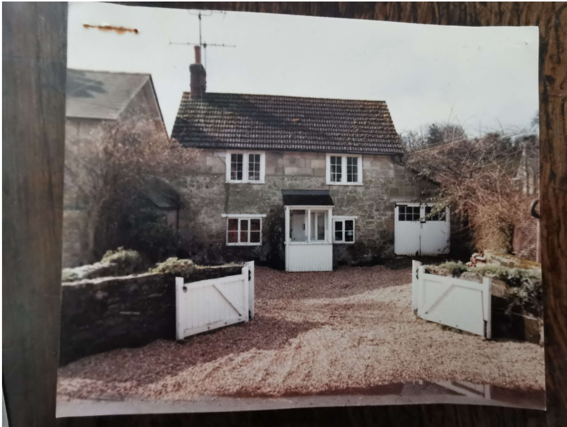
Photograph 04, Historic photograph showing previous porch to front elevation.
