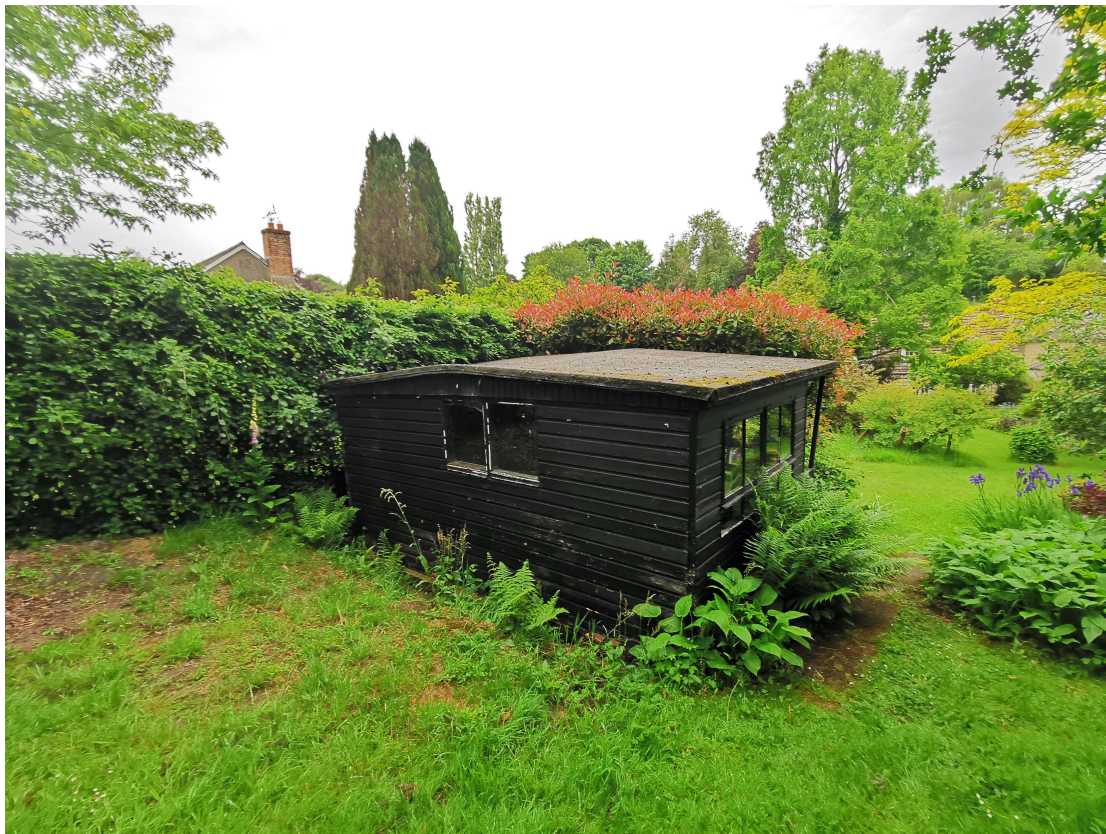
Photograph 03, Existing workshop to rear garden.
