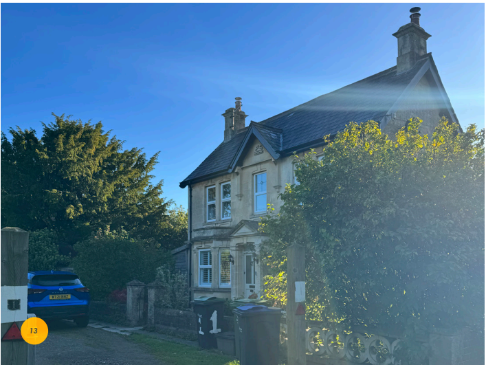
Fig 13. Side extension only visible when approaching the site curtilage
