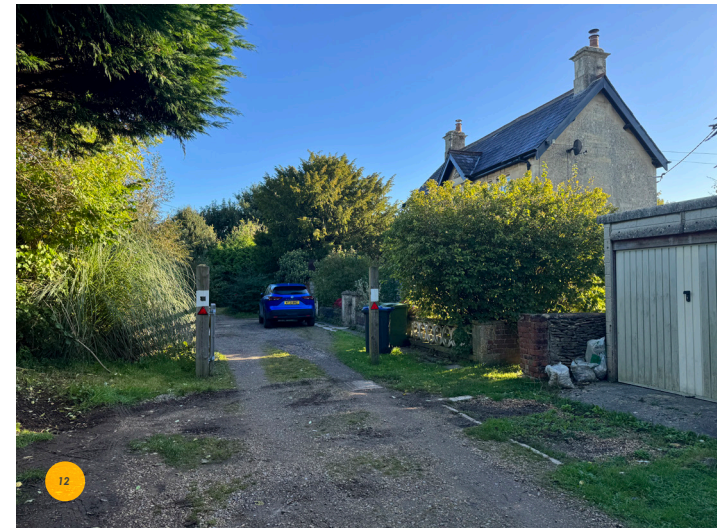
Fig 12. Photograph of existing condition, showing side lean-to extension obscured from view
