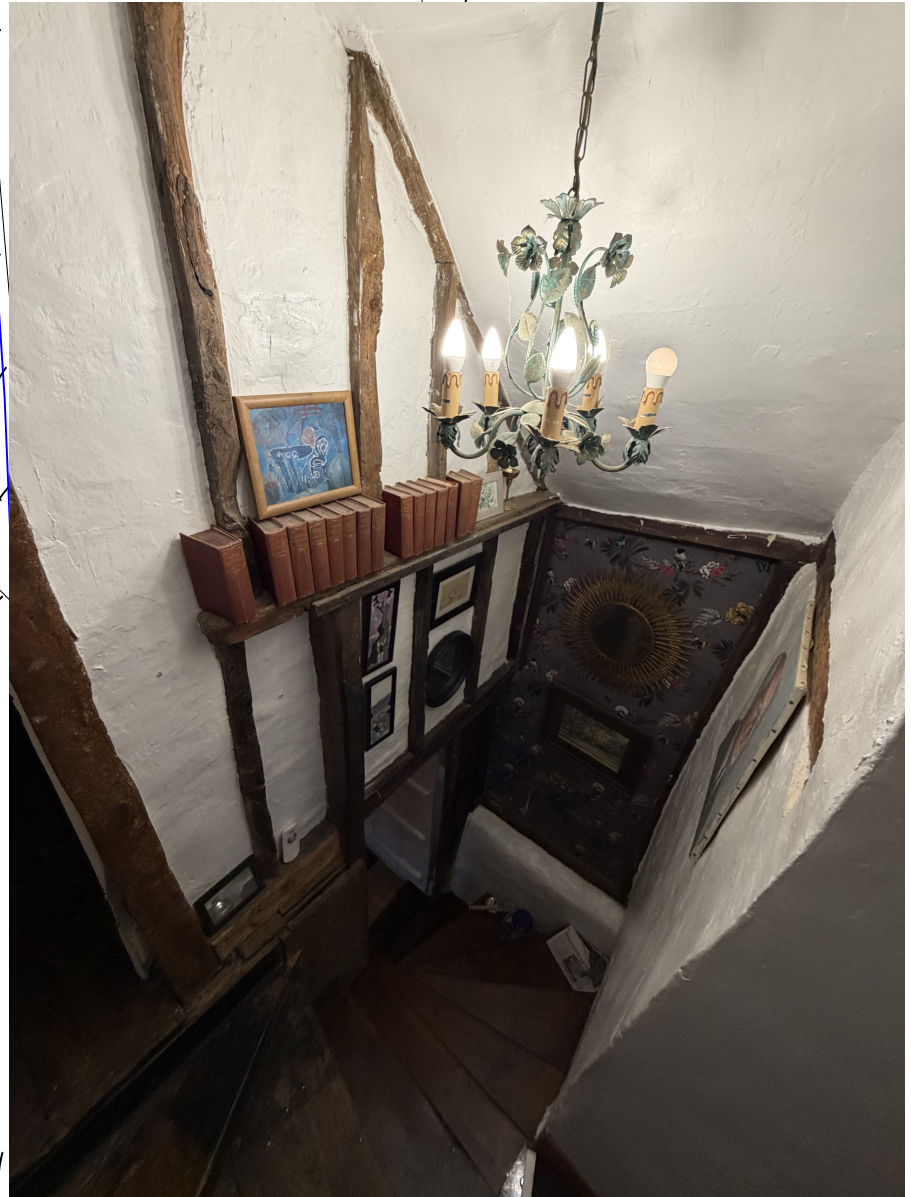
photo of existing stair
