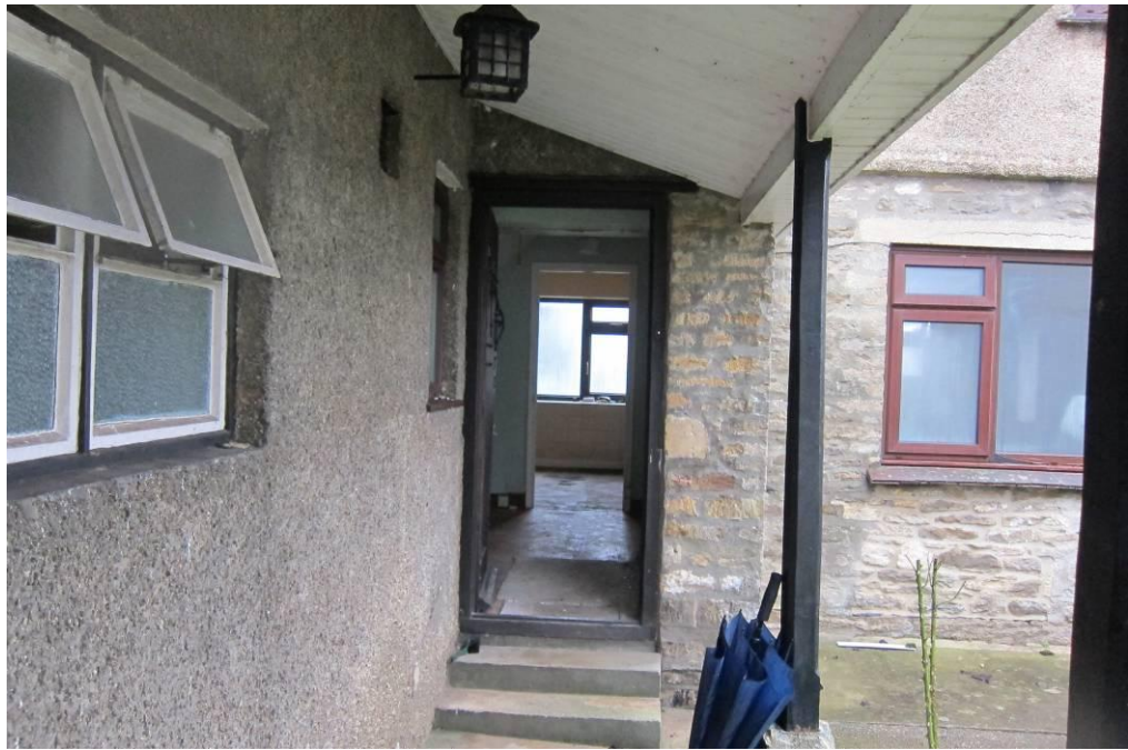
Fig 4. Porch and entrance
