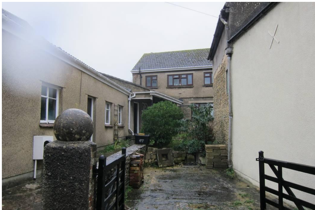
Fig 5. Parking and garage
