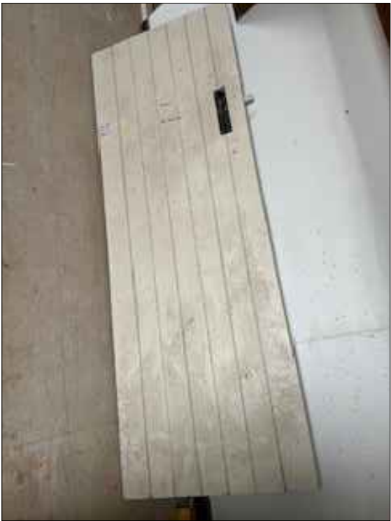
Front of the reclaimed boarded door- v joints Dimensions: 685mm (W) X 1940mm (H)
