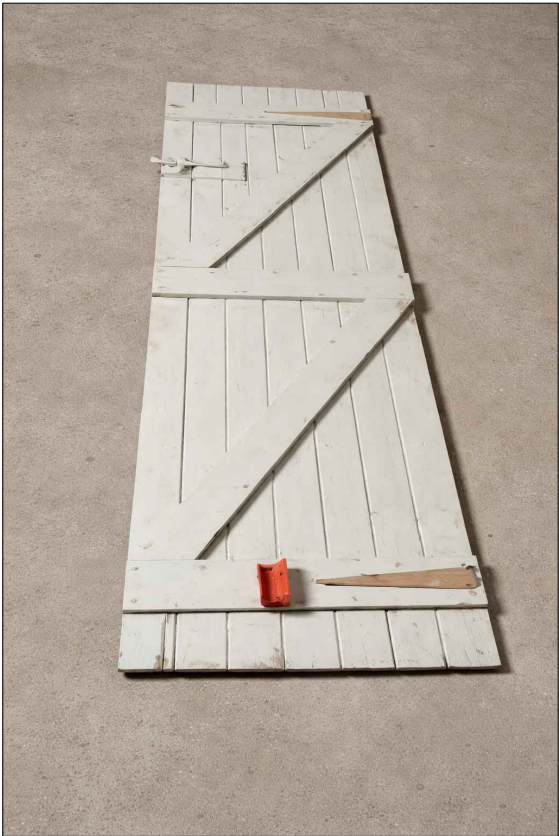
Rear of the reclaimed boarded door- Ledged and braced
