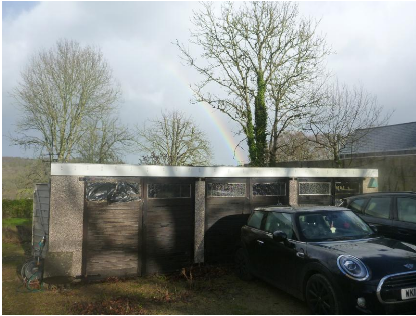
Fig 3: Doors on the southern face of the garage are kept closed and secured.
