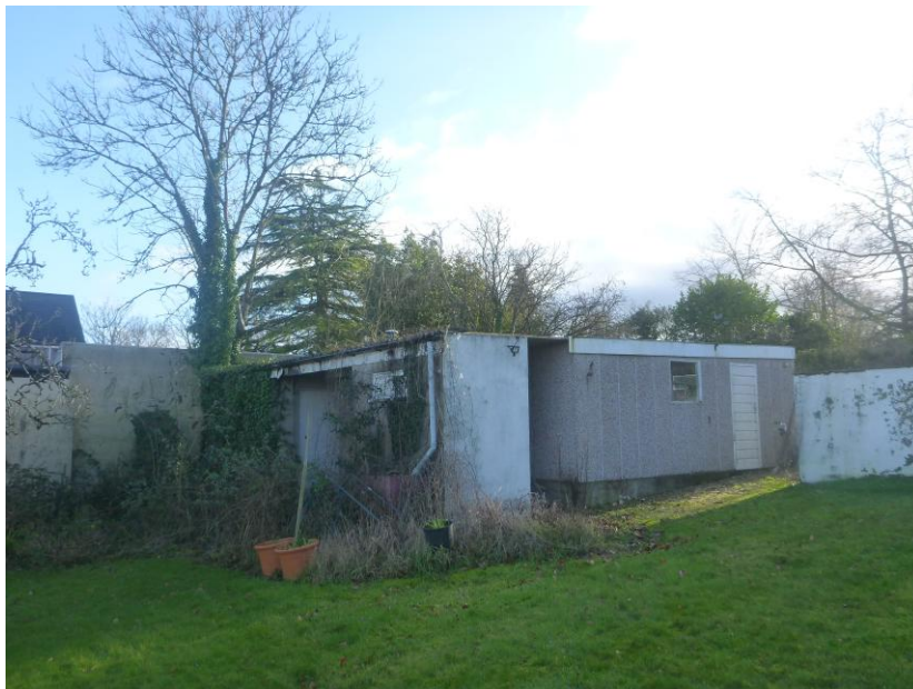
Fig 2: The garage at Coppice Dell.
