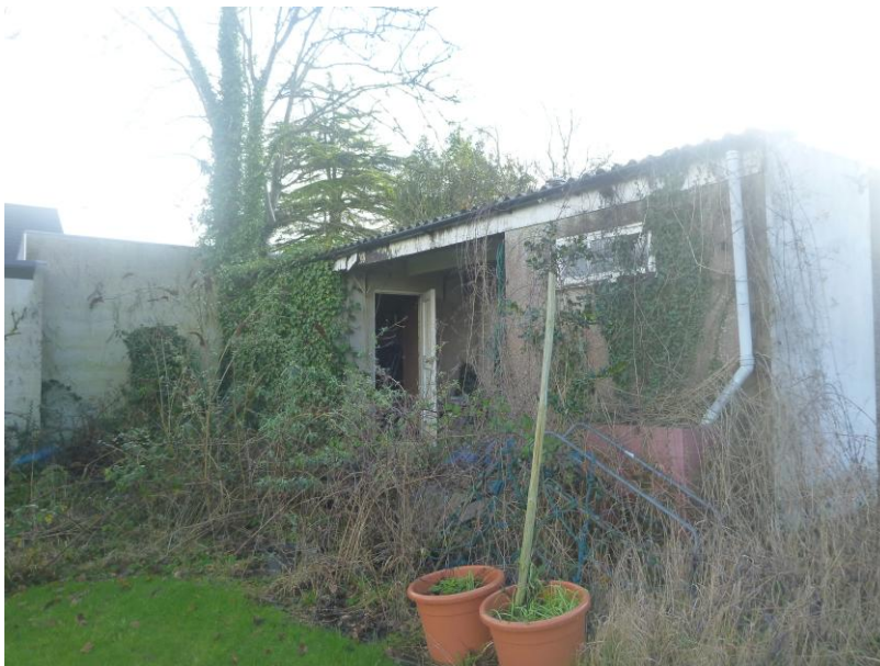
Fig 6: The rear of the garage is covered in ivy.
