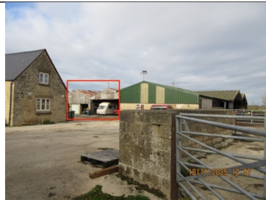
Photo 11. View towards the Site (highlighted red) from the south with the farmhouse in foreground
