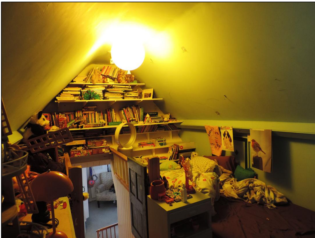
Photo 8 Steep narrow stair leading to Bedroom 3 within the eaves of the 1930s extension. The narrow room with restricted head space is currently not suitable for modern living.
