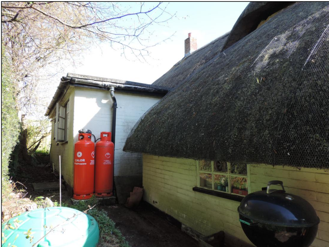
Photo 4 ESE facing view of north elevation of Ash Tree Cottage. Photo Date 25/03/2025.
