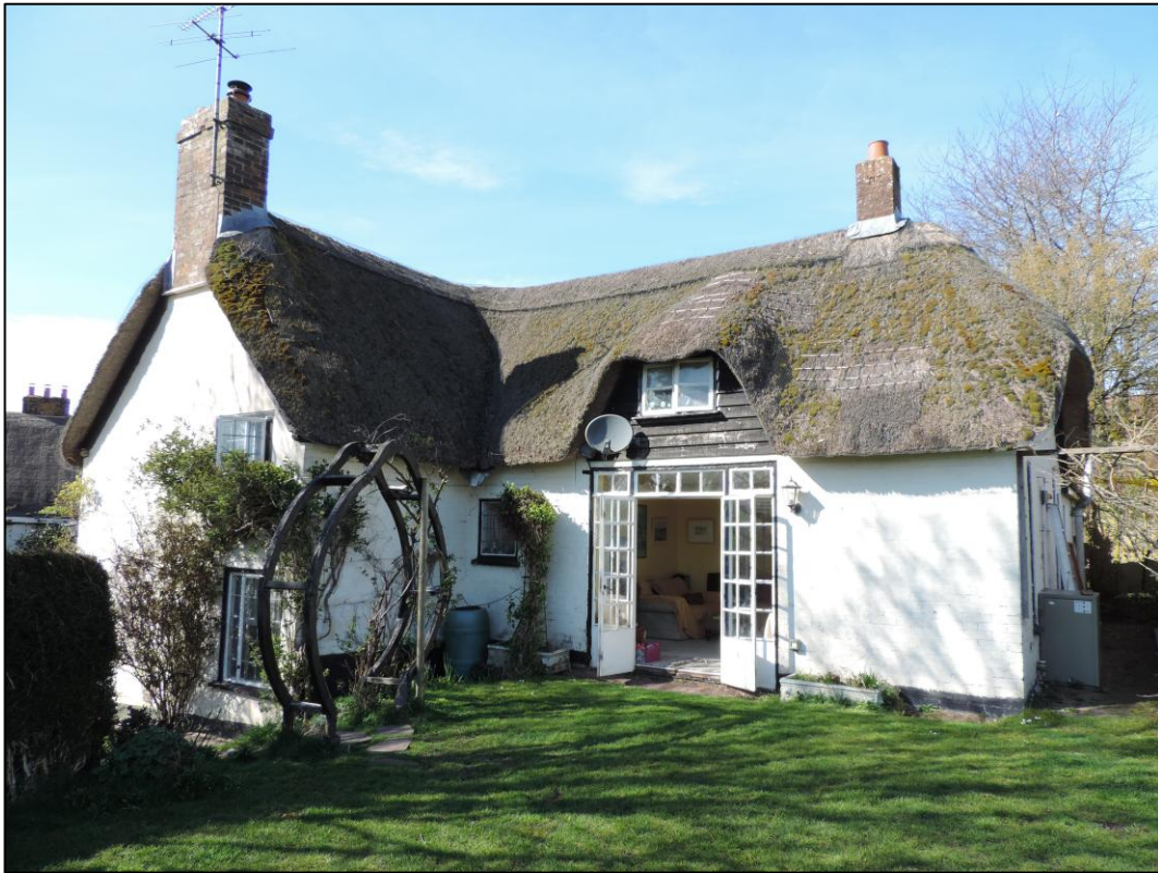
Photo 3 Northwest facing view of the south elevation of Ash Tree Cottage. Photo Date 25/03/2025.
