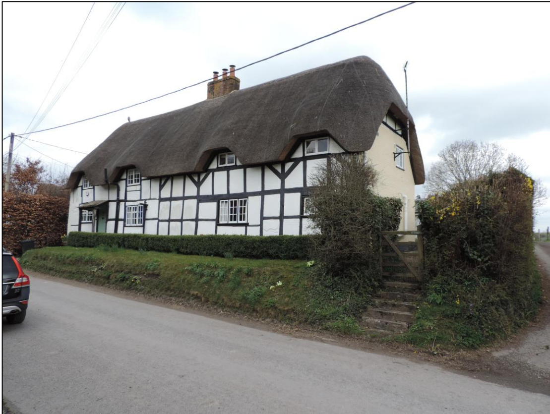
Photo 2 NNE facing view towards Priory Cottage (formerly Avon Cottage) from the high street, March 2025.
