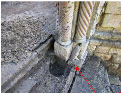
Column supported off riser of steps
