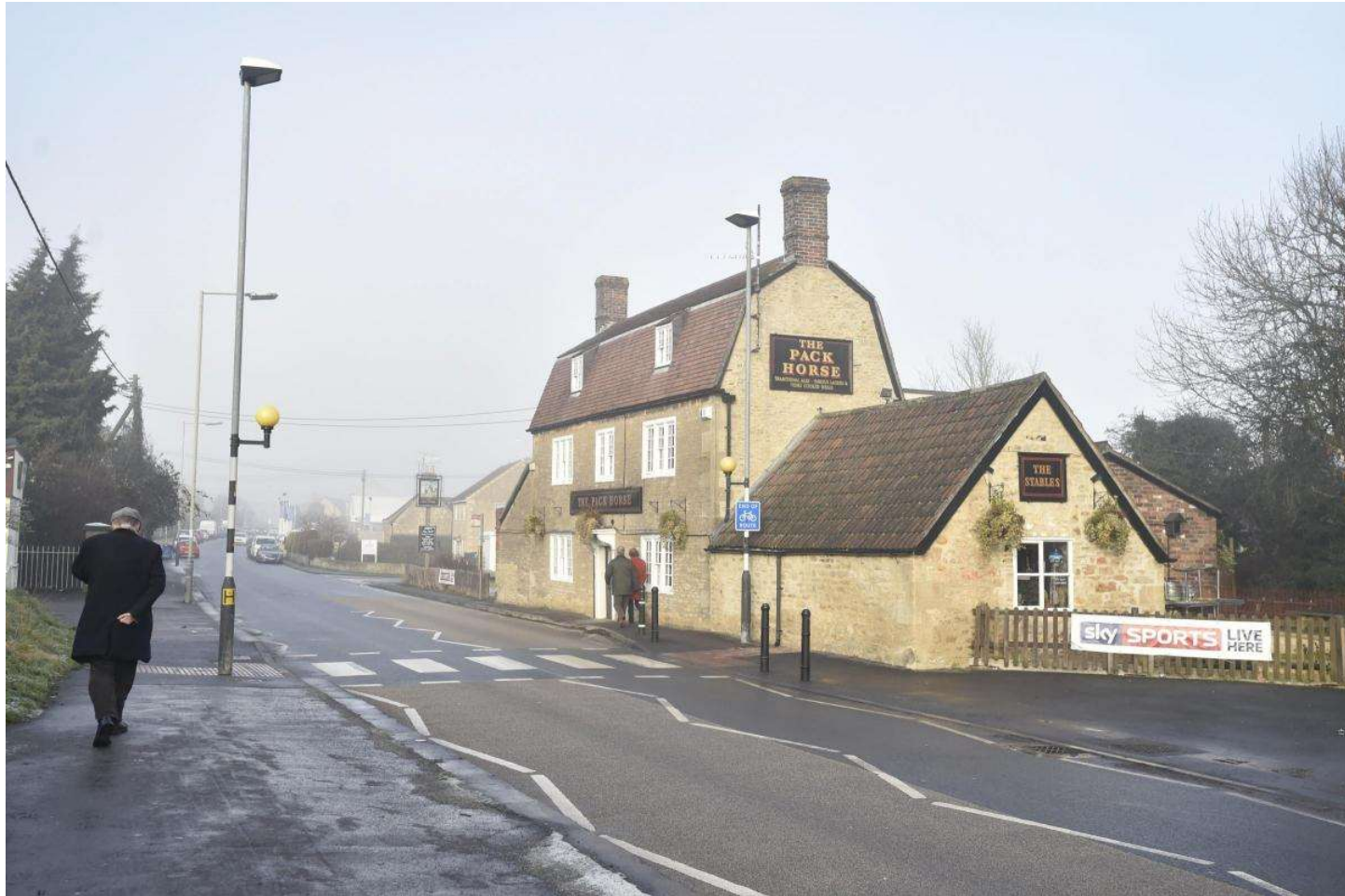
Figure 3.1 – Street view of The Pack Horse, 104 London Rd (Grade II Listed) – traditional hipped roof with dormers
