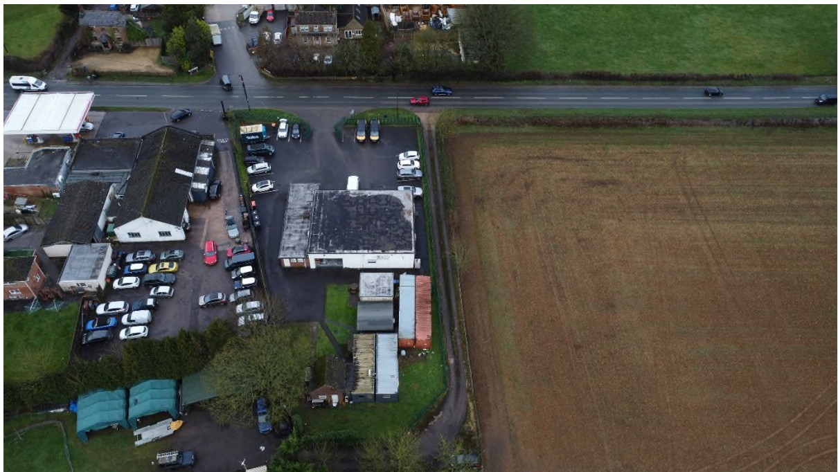
Plate 2 showing site conditions looking north
