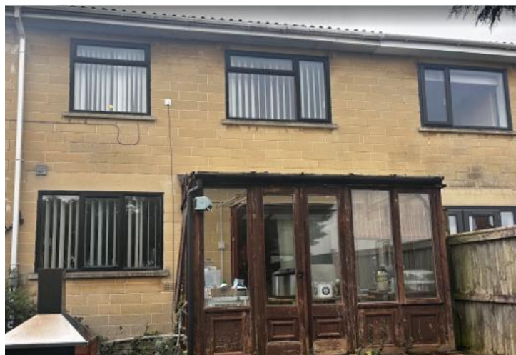
Rear elevation of No. 112 with the patio doors of No. 114 shown adjacent
