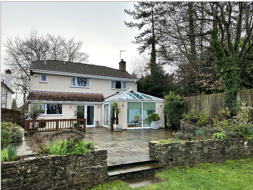
Figure 4: Large paved surface to rear of property. T5 is located in a shrub border beyond a retaining wall.
