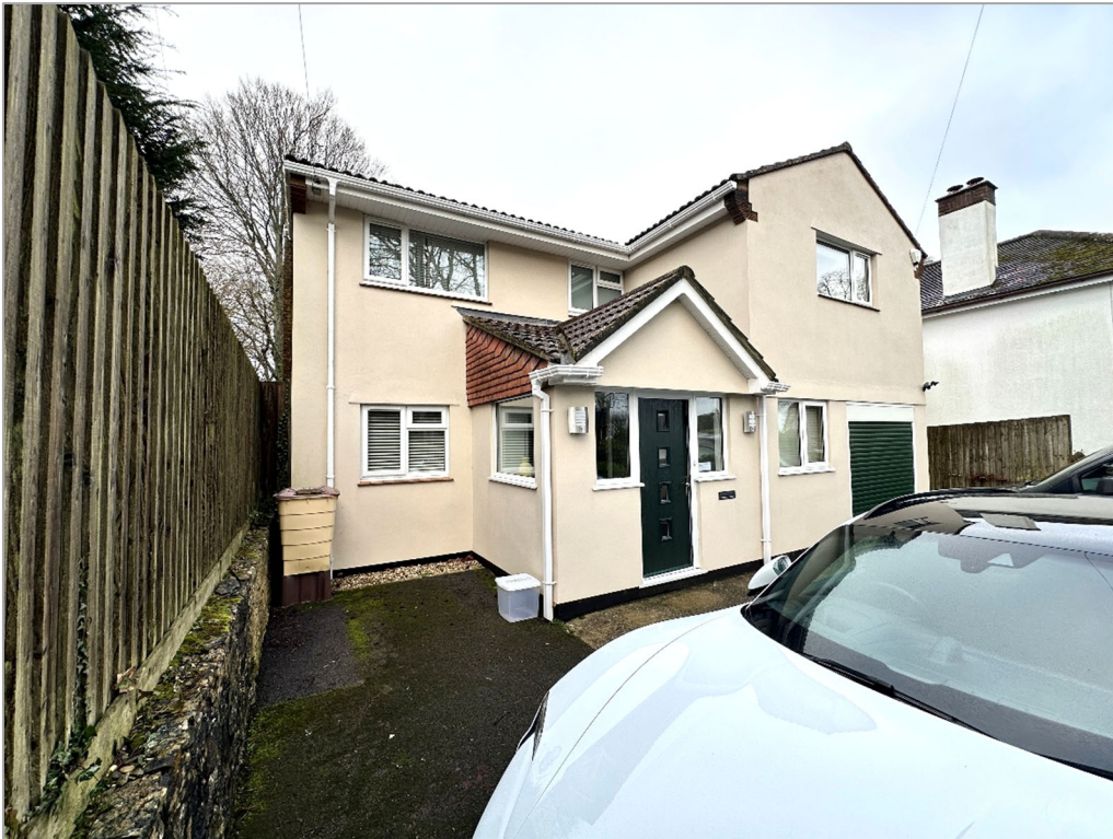
Figure 3: Front of house. 850mm high retaining wall located to the left of the photo.
