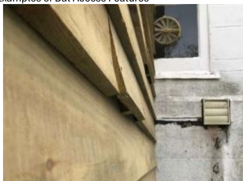
Example of cladding based crevice roost
