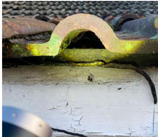
Plate 12: Side porch triple roman tiles and example of a gap which could be used by roosting bats for access
