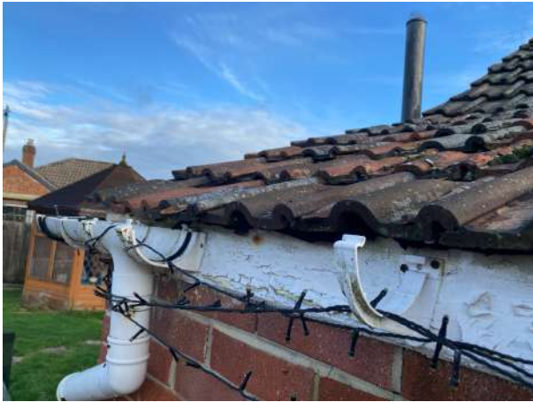
Plate 12: Side porch triple roman tiles and example of a gap which could be used by roosting bats for access
