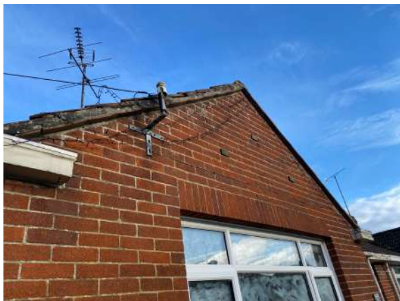
Plate 13: Gable end of bungalow with crevices in mortar under tiles
