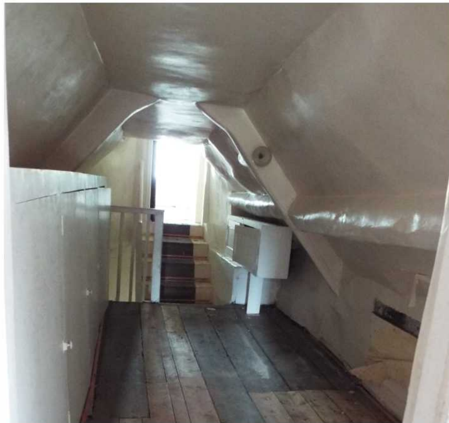
Cell 'E' 17th - 18th C roof structure
