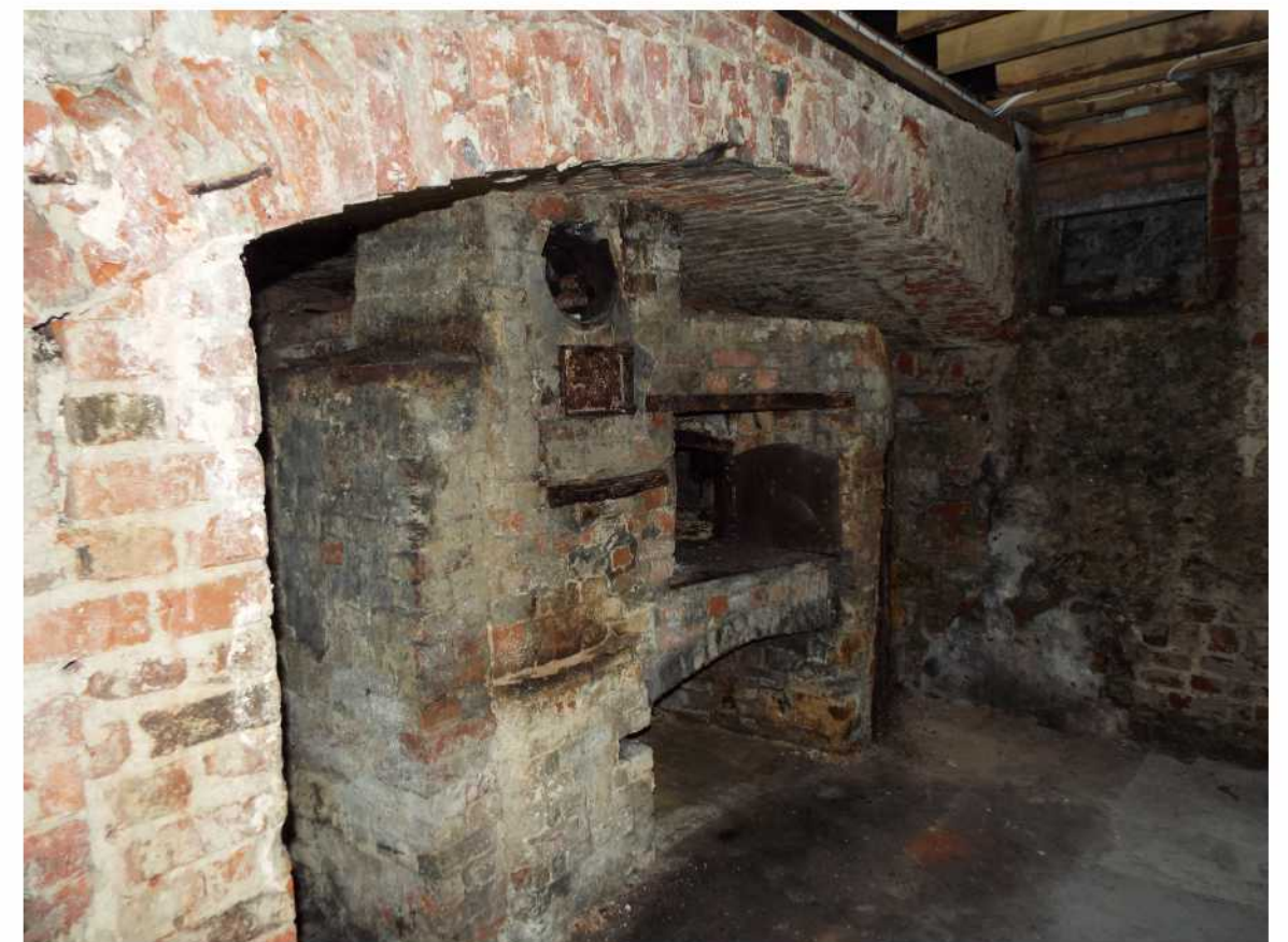
Cell 'H' oven ensemble in cellar
