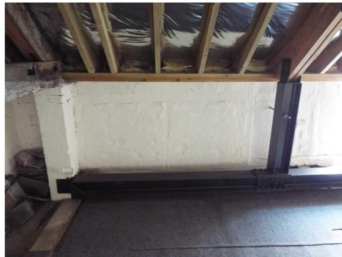
Cell 'B'. Roof structure.
