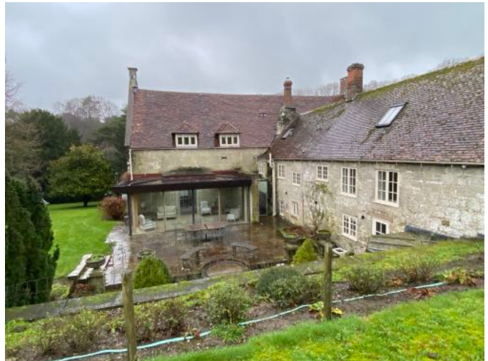
Image 14: View of the northern aspects of both roofs from above the pool room.
