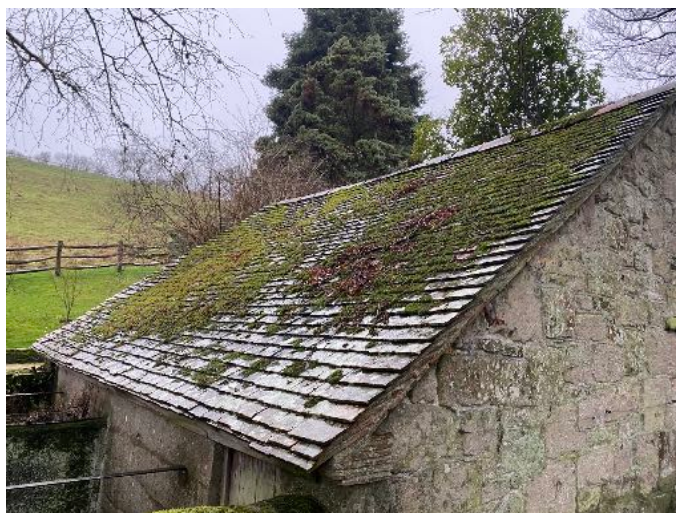
Image 26: Southern roof of B3.
