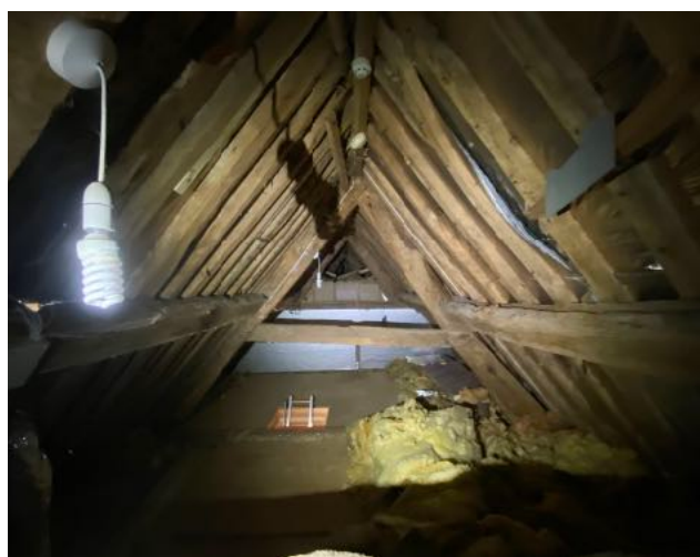
Image 20: View from southern aspect of L1 facing northward.
