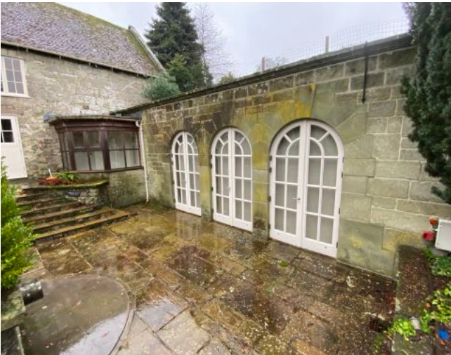
Image 13: Front side of underground pool.
