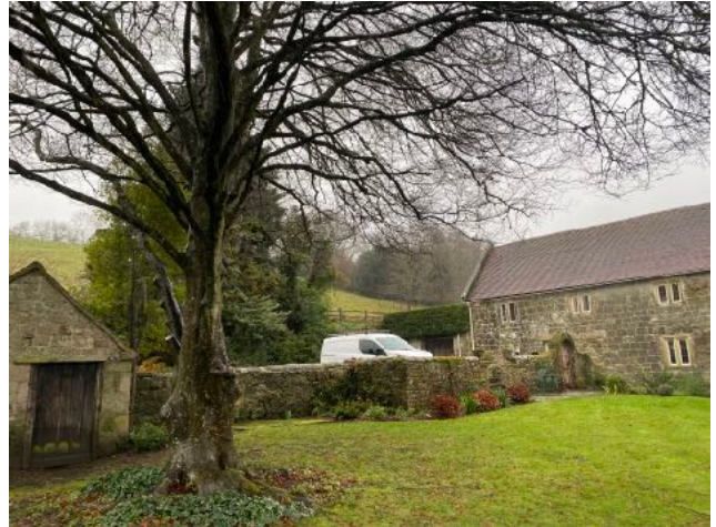
Image 2: Driveway, small out house (B3) and large beech tree on the southern aspect of the site.
