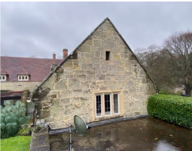
Image 15: Western gable end with meshed open window.
