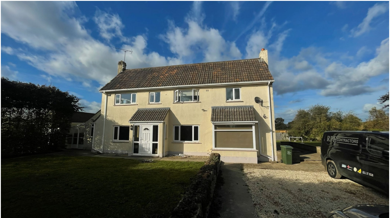
Photograph of existing principal elevation February 2025
