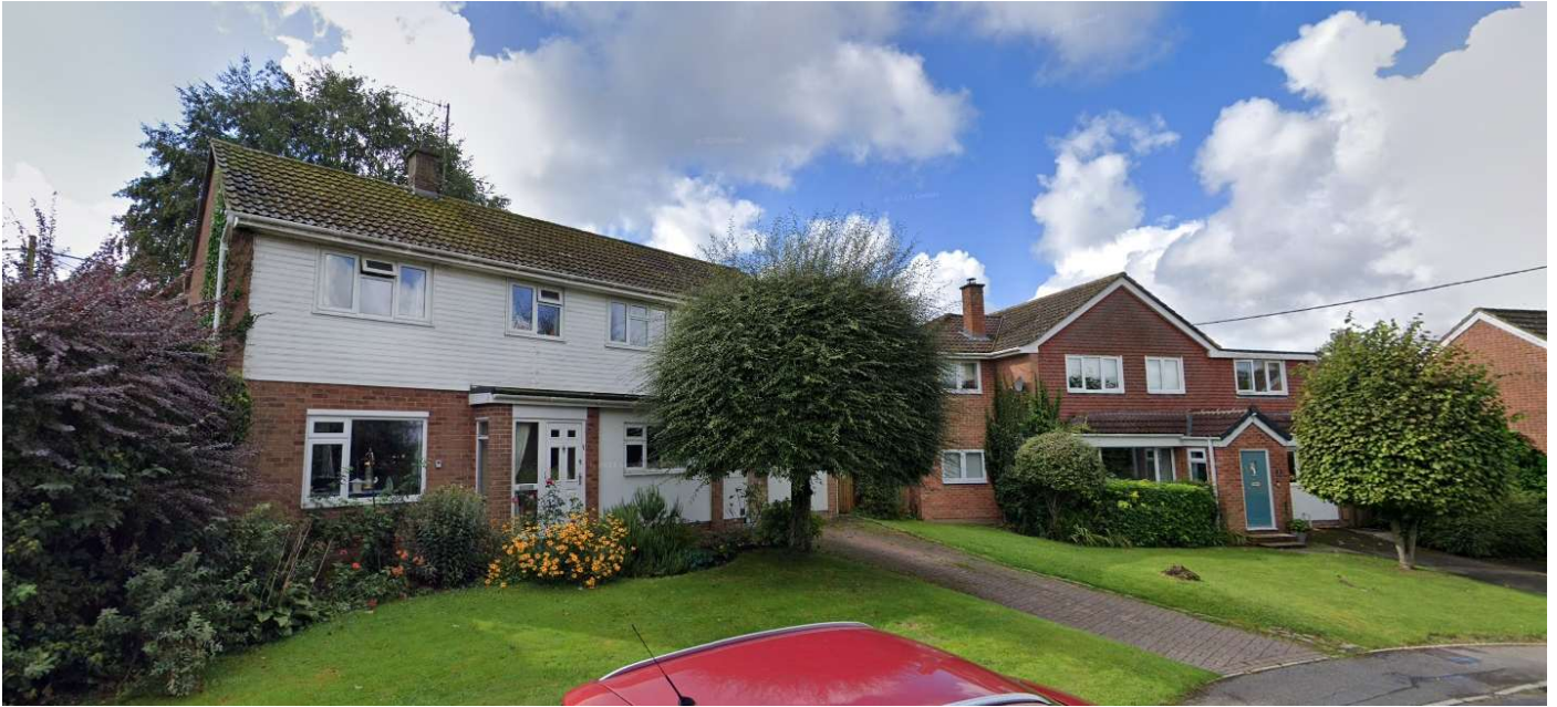
Fig 3.3 Photograph of property types in Elcot Close (Google maps)
