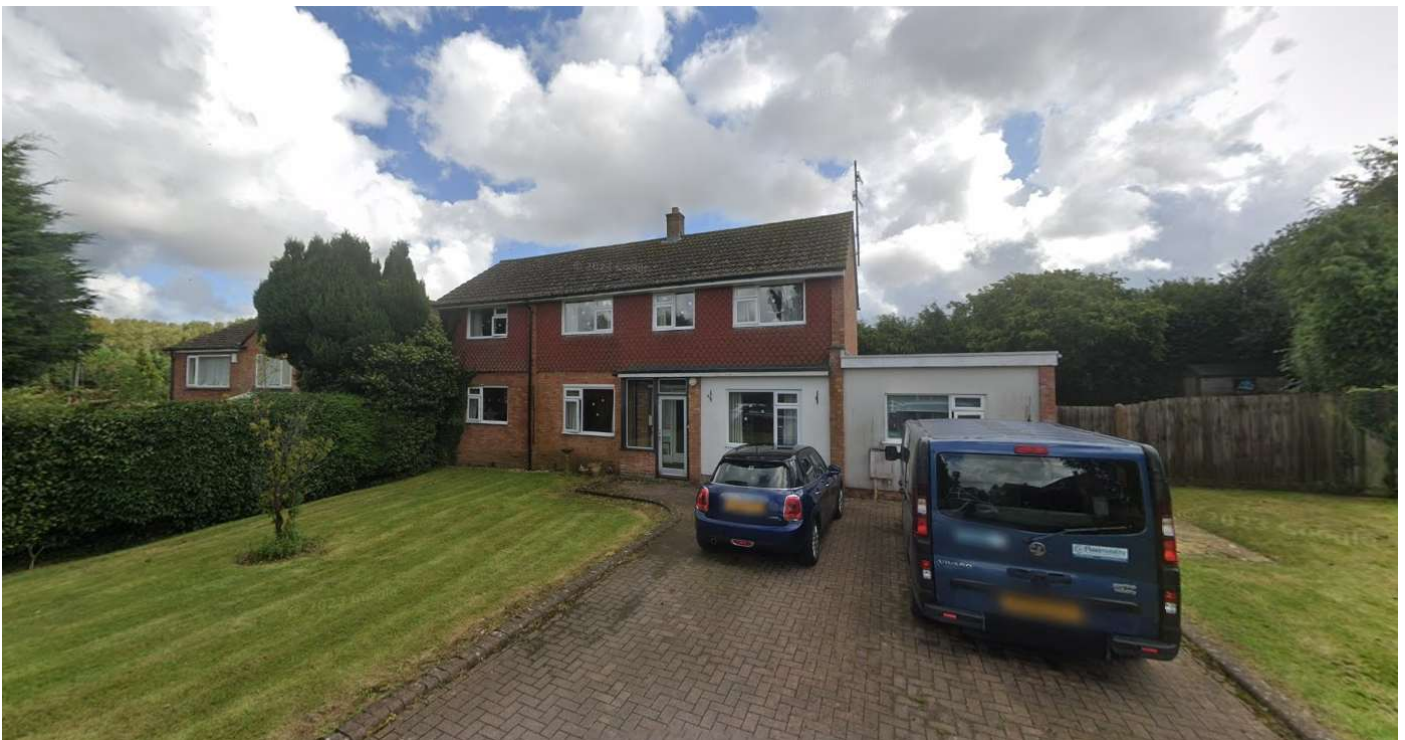
Fig 1.0 Photograph of 5 Elcot Close (Google maps)
