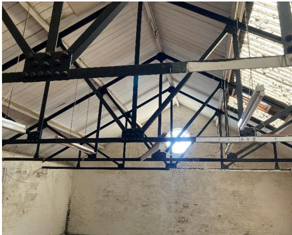
Figure 6 - Loft space of Block B.
