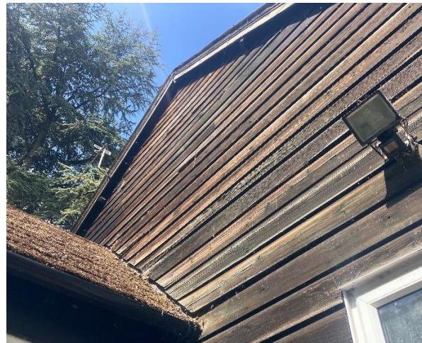
Figure 14 - Scott's Gym, south side.
