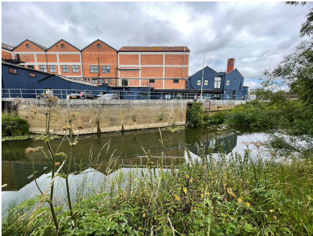
Photograph 4: View towards the north across the River Avon, showing the concrete retaining wall, sluice structure and Units B, C and G.
