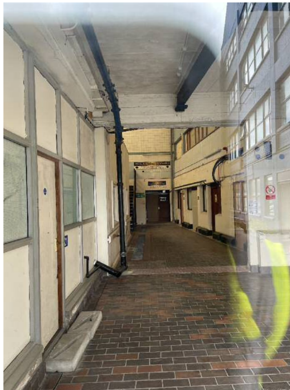
Photograph 12: View towards the east of the internal section of Unit D proposed for demolition.
