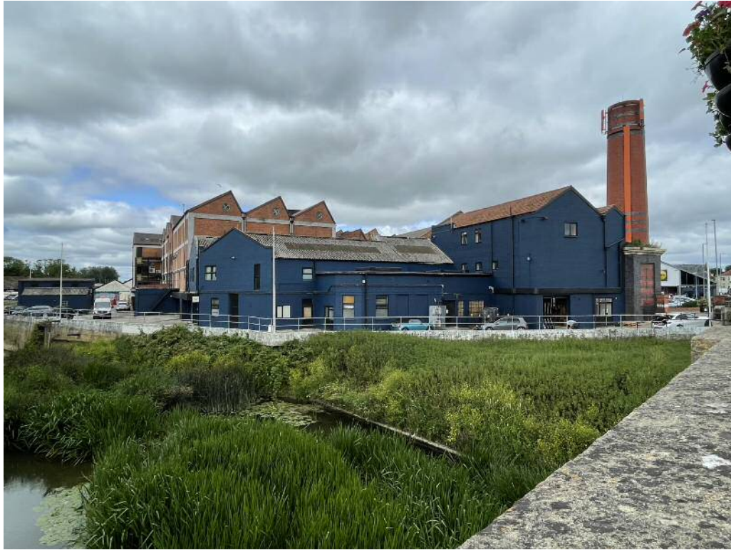
Photograph 3: West facing view of the eastern end of the site (Units F, G, 15 and electrical substation).
