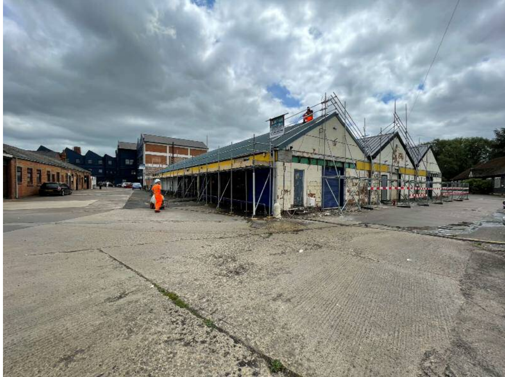
Photograph 10: View towards the southeast of Unit 3 and 7 – 11 and the former gym/scout hut.
