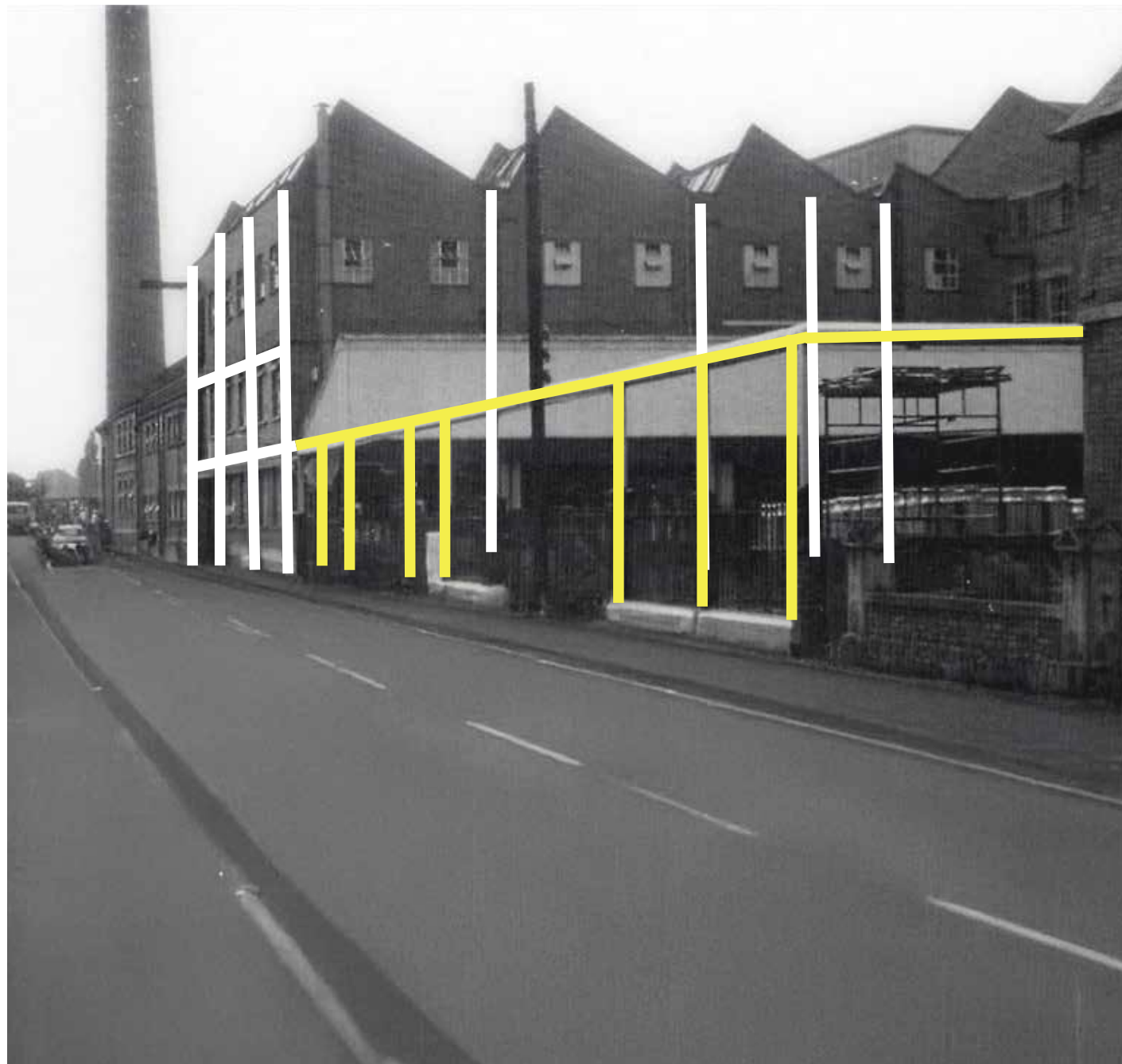
New Broughton facade and structure over northern car park c.1968
