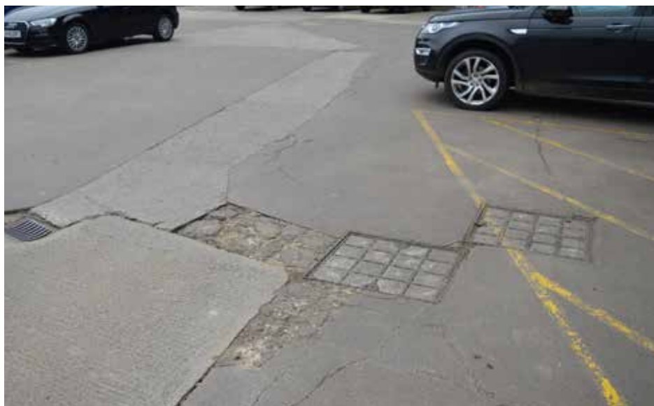
6 - Layers of existing surfacing
