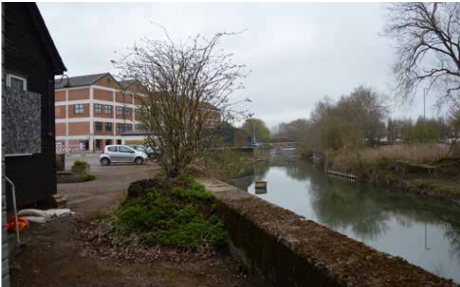
1 - Concrete flood wall without railing
