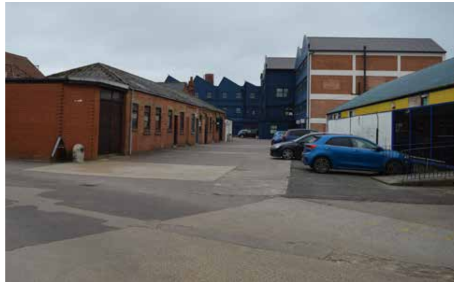
4 - Mix of concrete and tarmac surfaces with localised fractures and subsidence
