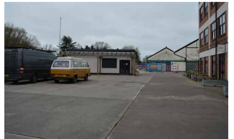
8 - Large cast in situ concrete slabs
