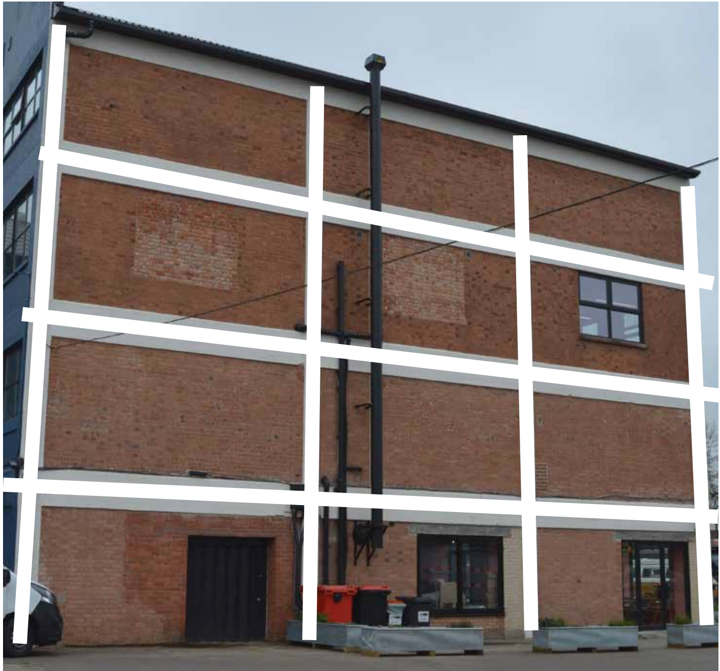
Block A facade
