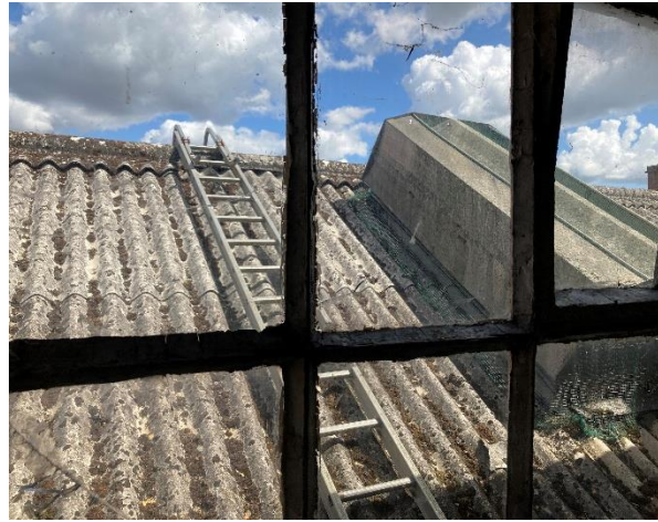
Figure 11 - The roof of the building
