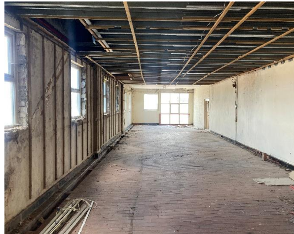
Figure 7 - Top floor of Block D.
