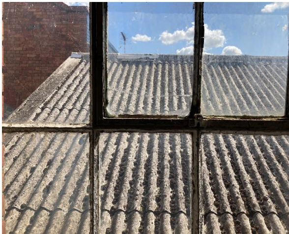
Figure 11 - Roof of the main building.
