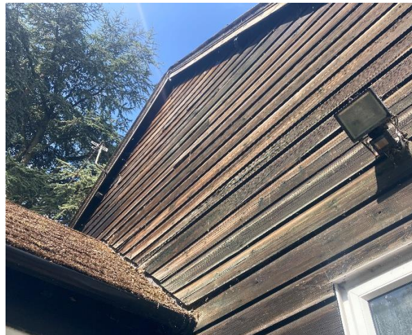
Figure 14 - Scott's Gym, south side.
