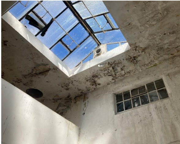
Figure 10 - Top floor/loft space of Block D
