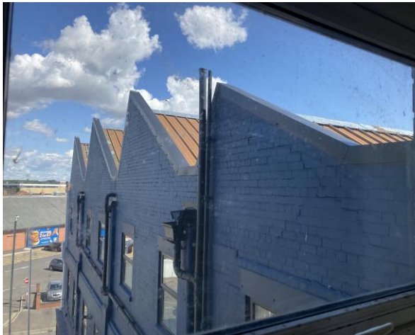
Figure 4 - The external of Block D. Brickwork all intact, barge board flush with no gaps. The rest of the main buildings had the same external conditions.
