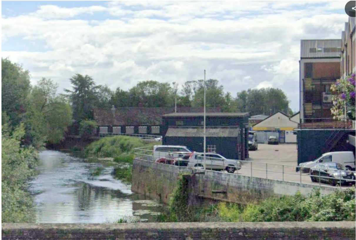
Figure 3 - Photo taken from google street-view, showing the height of the embankment separating the site from the River Avon. © 2025, Google.
