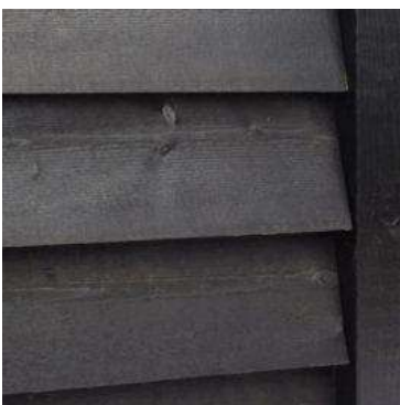
Dark stained horizontal weatherboard cladding
