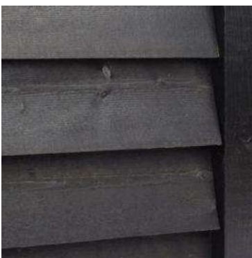
Dark stained horizontal weatherboard cladding
