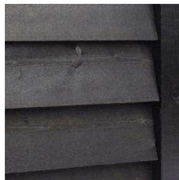
Dark stained horizontal weatherboard cladding
